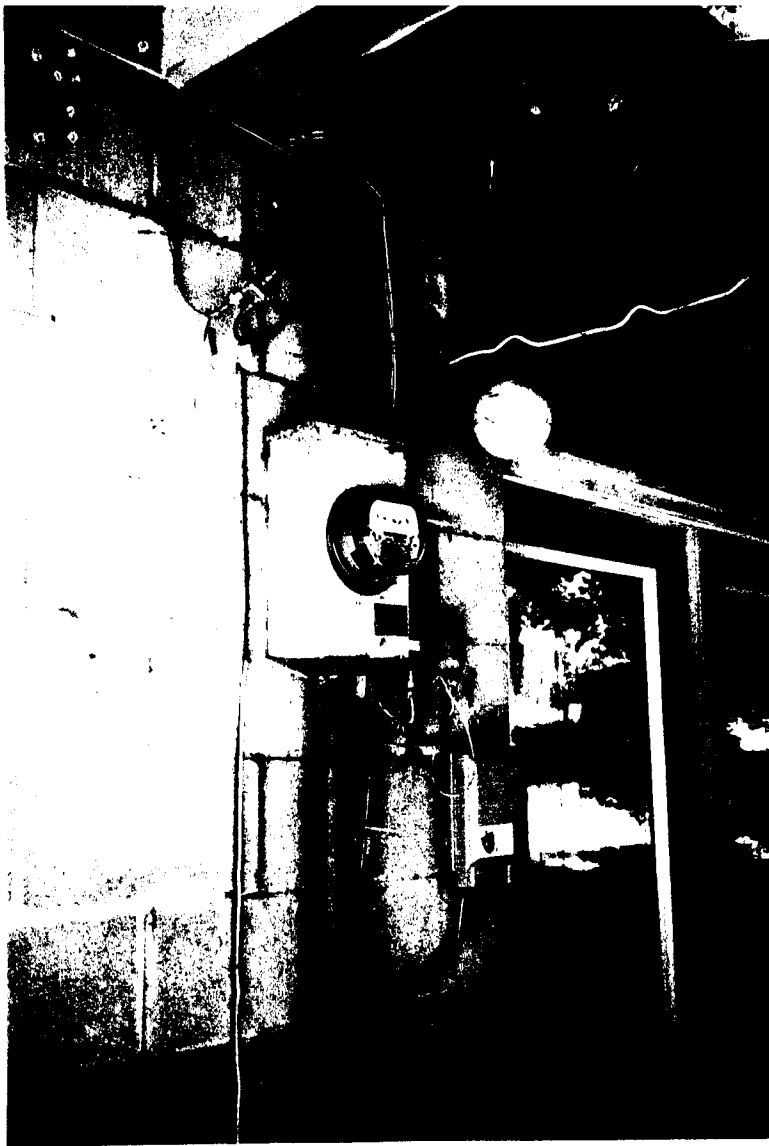
bundled phone, cable and security wires - note multiple wires running through eaves
