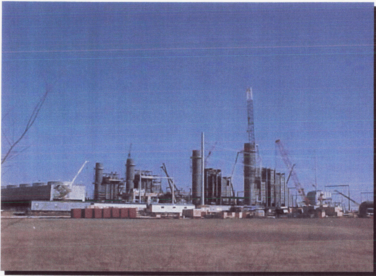
View of Paris Project from SW Corner 02/08/2000
