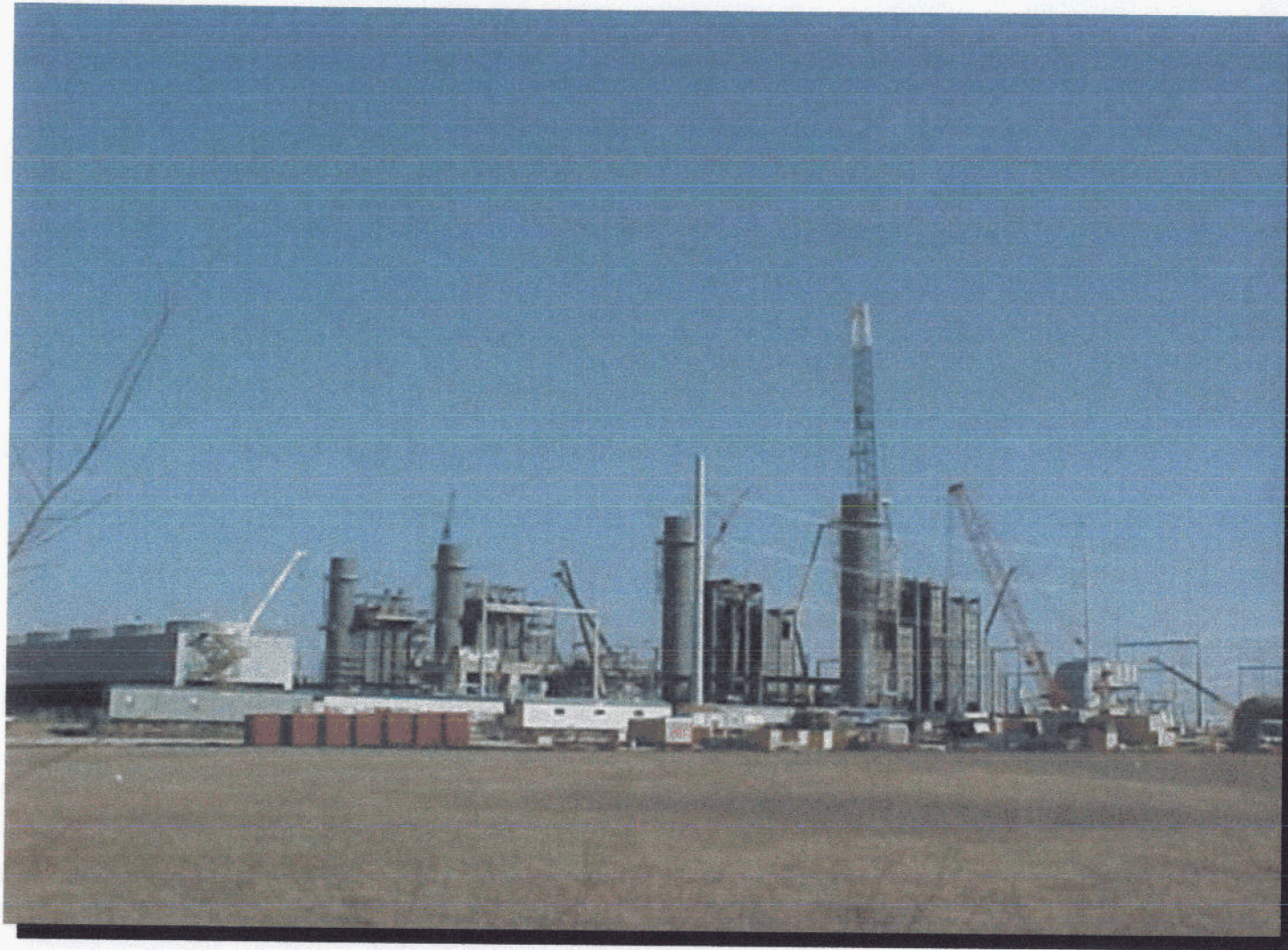
View of Paris Project from SW Corner 02/08/2000
