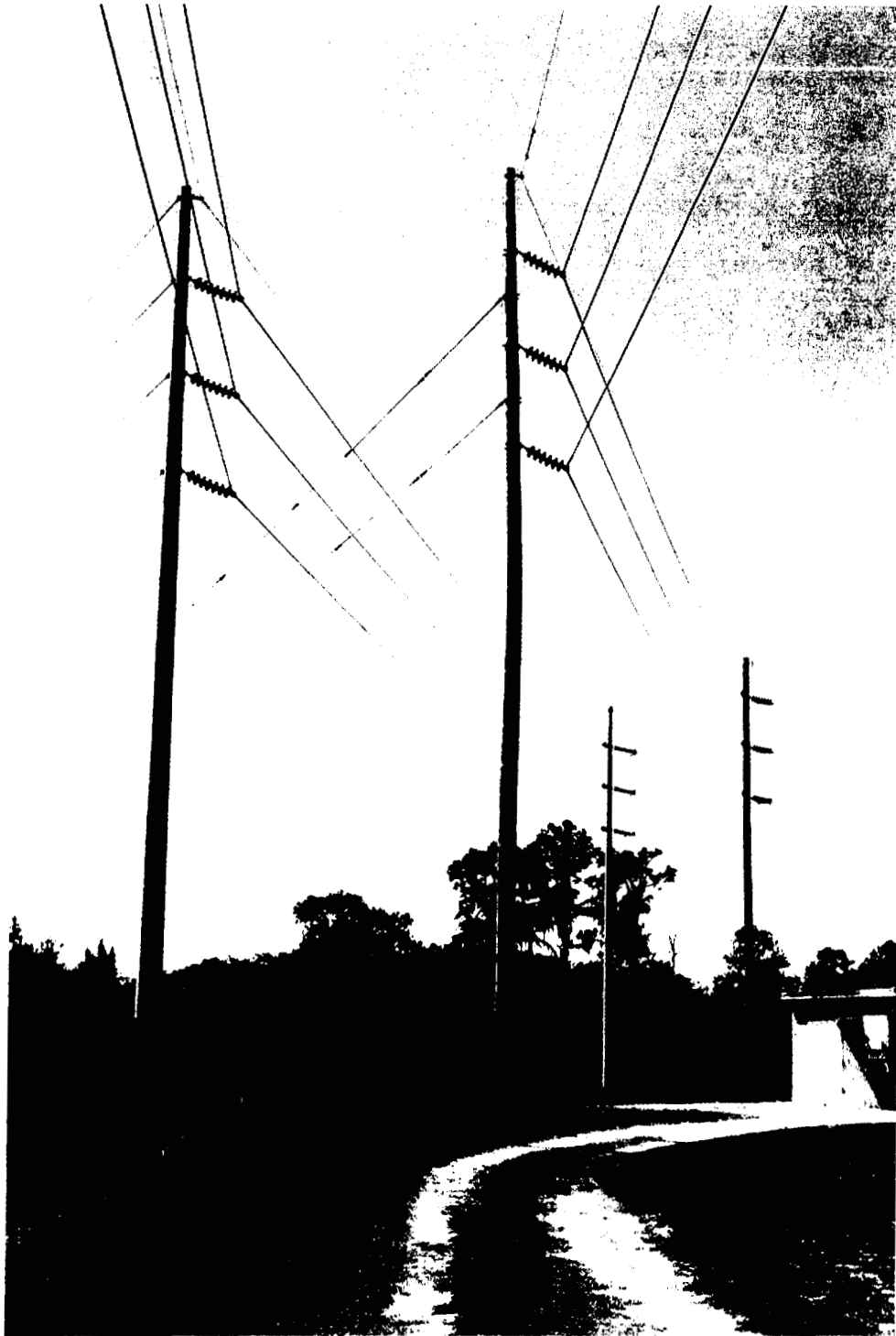
Picture 12: Typical single pole wood and concrete angle structures
