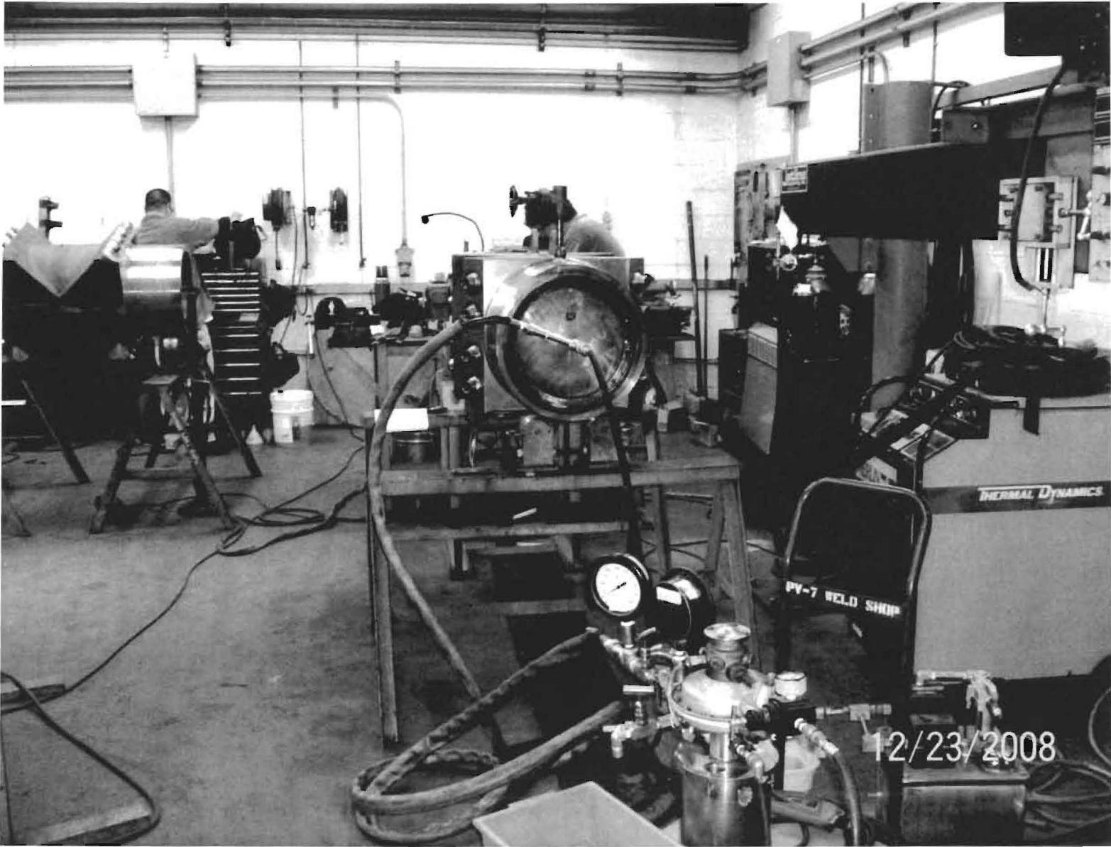
Docket No. 090009-EI Ultrasonic Flow Metering Hydrostatic Pressure Testing of the System Exhibit RSK-4, Page 1 of 1
