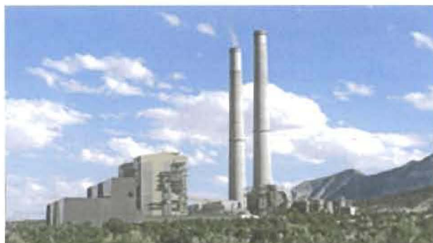
PacifiCorp's Huntington Power Plant in Huntington, Utah
