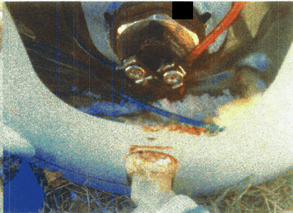
2212 hot water heater – example of how crystals fill up tank making it even hard to flush them out.
