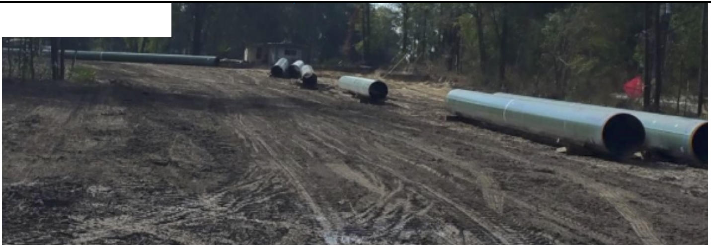
Pipeline ready for installation in Newberry, Florida. Critics say construction could permanently destroy nature preserves and aquifers. Credit: Jesse Hughes
