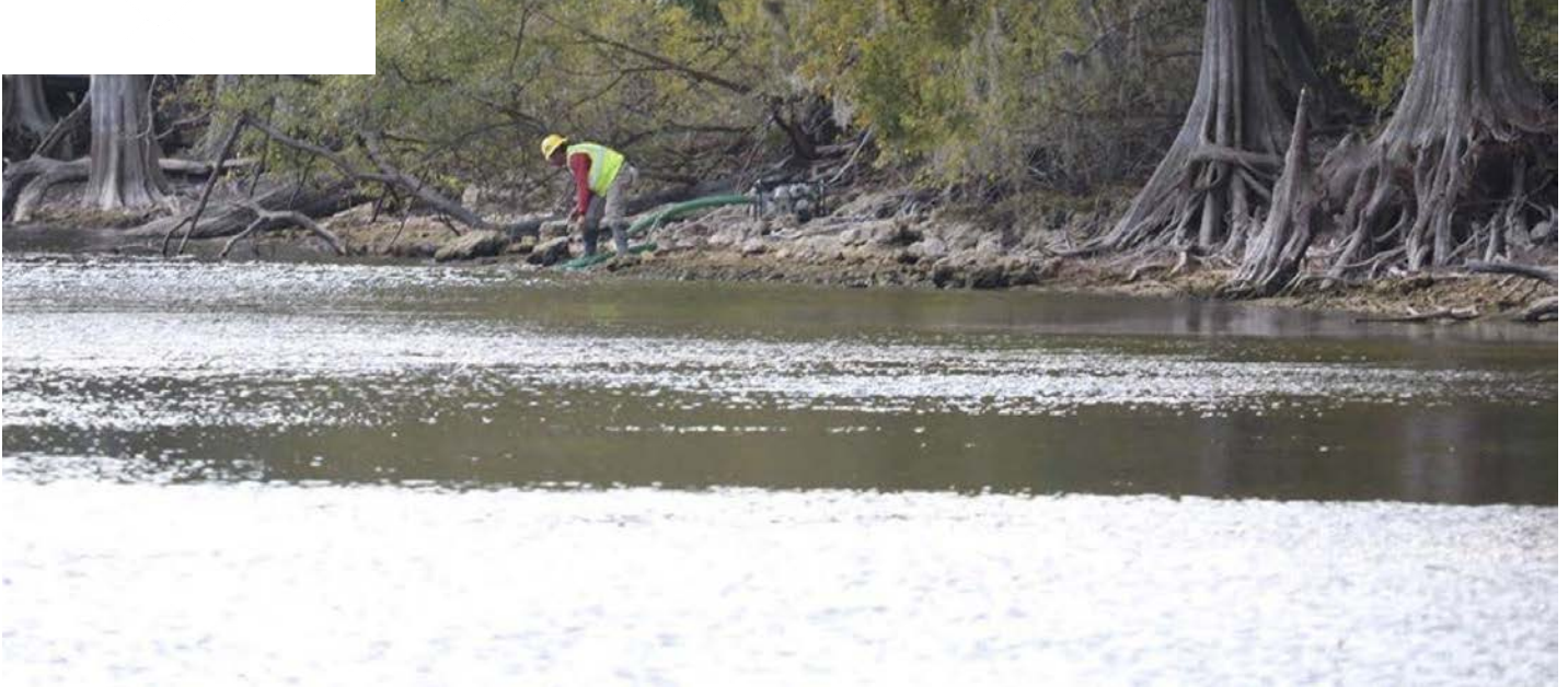
A Sabal Trail pipeline worker in central Florida. The pipeline will run through conservation areas, under rivers and near springs. Credit: Merrilee Malwitz-Jipson
