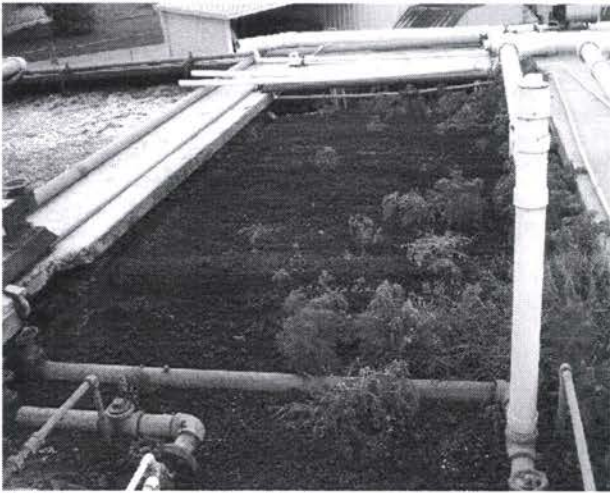
Solids and vegetation in the west clarifier.
