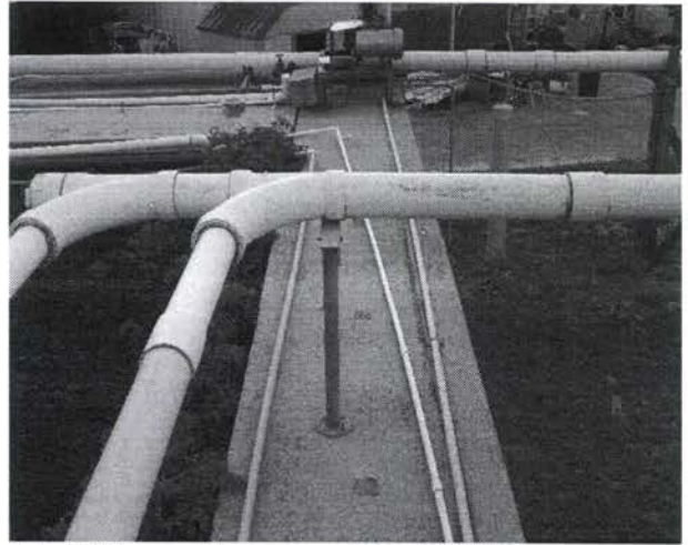
Trip/fall hazards on top of the WWTF.
