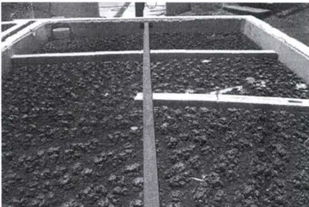
Solids in the north chlorine contact chamber (CCC).
