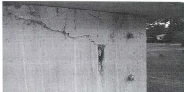
Cracks/leaks in the wall of the aeration basin.
