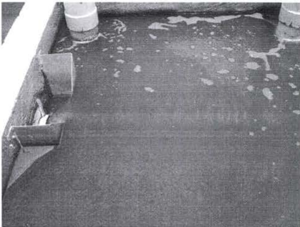
Excessive solids in the final effluent.
