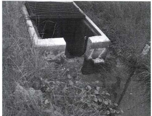
Discharge to the Wekiwa River via this drop inlet.
