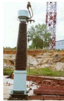
Figure 34. 400-kV Current Transformer
