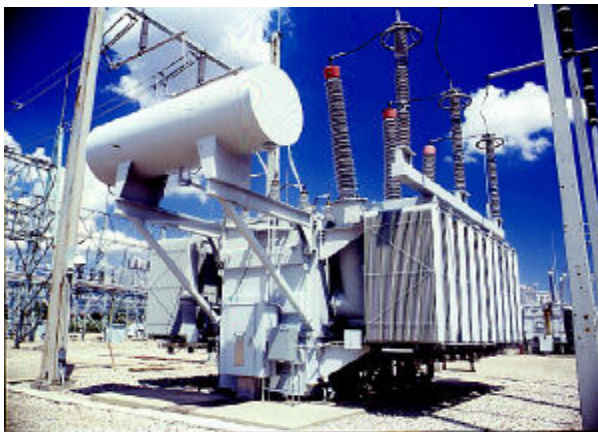
Figure 35. Power Transformers
