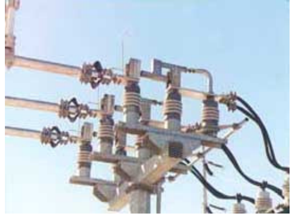
Figure 38: Air Circuit Breaker
