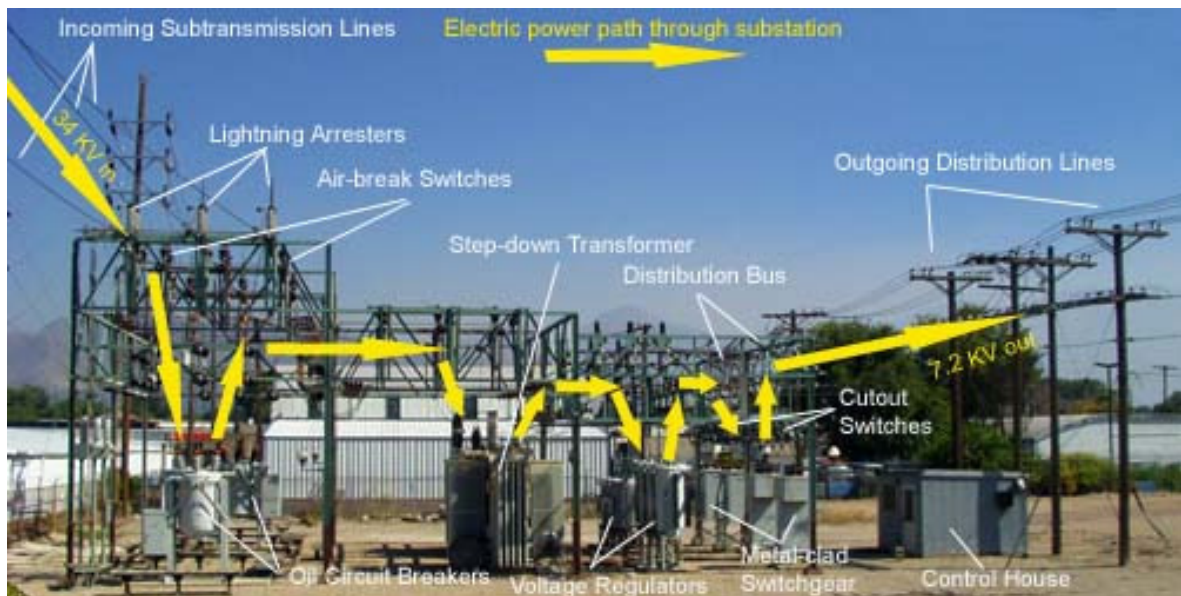
Figure 30. Transmission Substation
