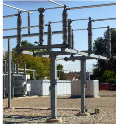
Figure 40. Circuit Switches
