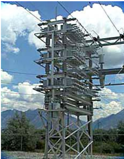
Figure 39. Capacitor Bank
