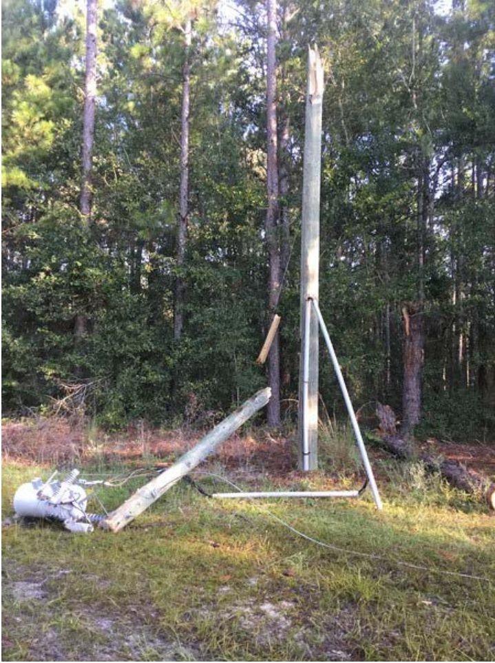
Example of a broken pole. SVEC's broken pole count from Hermine was 70.
