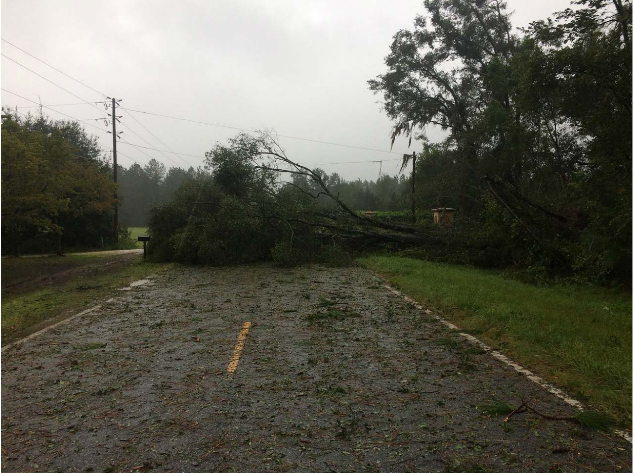
Example of tree damage that made many roads impassable for power restoration crews.
