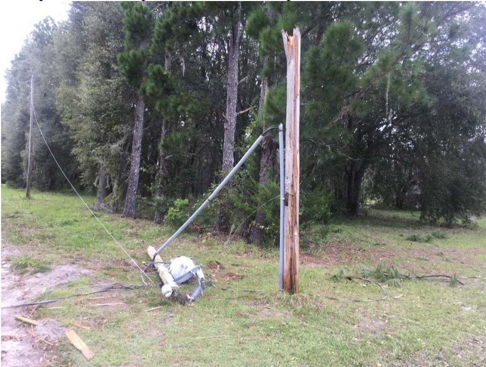
Example of a broken pole. SVEC's broken pole count from Irma was 240.
