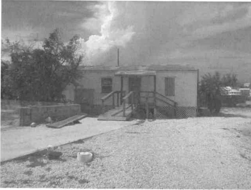
Photo 1. KWRU office building on day of inspection
