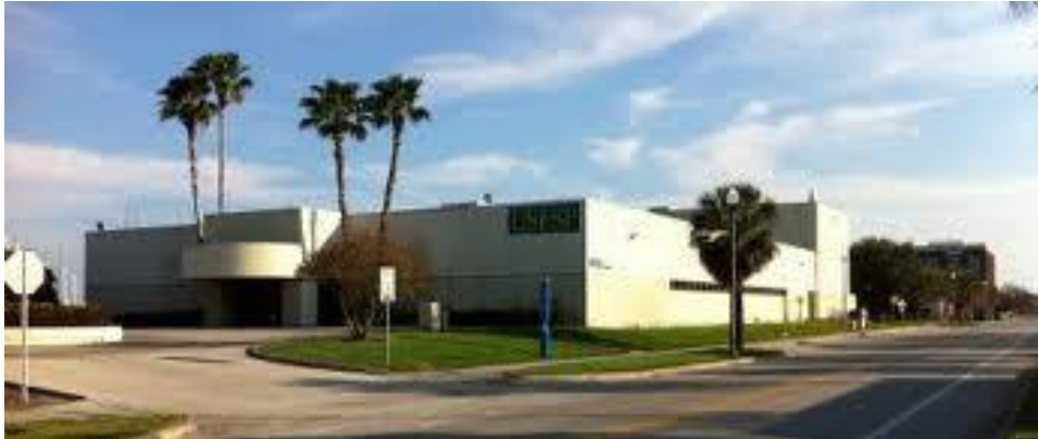
Figure 3. USF Harbor Hall Exterior View.
