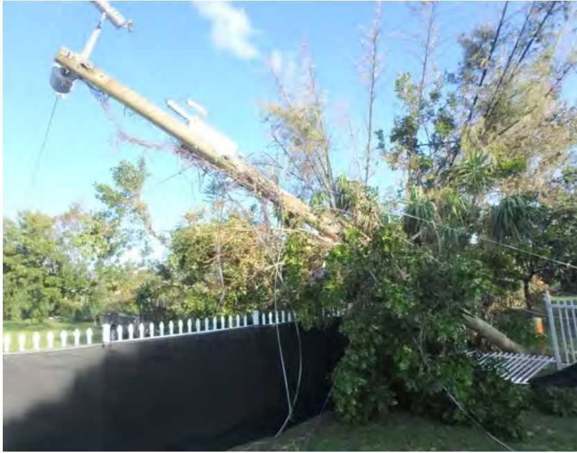
A power line is damaged during Hurricane Irma. (Photo: Courtesy of LCEC Archives)
