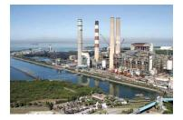
Big Bend units 1-4 are four (4) pulverized coal-fired steam units equipped with desulfurization scrubbers, electrostatic precipitators, and Selective Catalytic Reduction (SCR) air pollution control systems. Big Bend CT 4 is one (1) aero-derivative combustion turbine that entered into service in 2009 and can be fired with natural gas or distillate oil.
