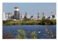
The station operates one (1) integrated coal gasification combined cycle unit and one (1) natural gas-fired combined cycle unit. Polk Unit 1 is an integrated gasification combined cycle (IGCC) unit fired with synthetic gas produced from gasified coal and other carbonaceous fuels. This technology integrates state-of-the-art environmental processes to create a clean fuel gas from a variety of feedstock with the efficiency benefits of combined cycle
