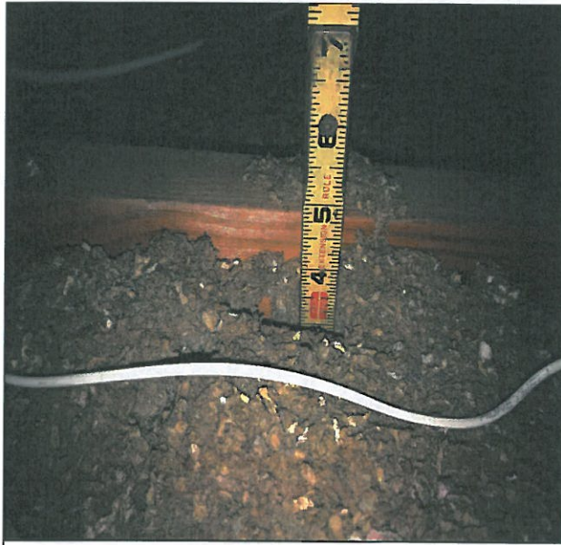
Approximately 4"-5" blown insulation (R-10).
