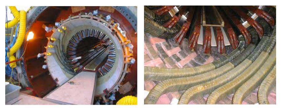
There is no practical method to inspect many areas of the winding for 'termite' activity, most of which may be under the top layer of the bar and thus invisible even if it was possible to inspect the whole winding
