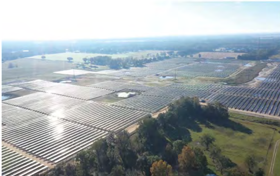
FIGURE 3.7 Trenton Solar Site
