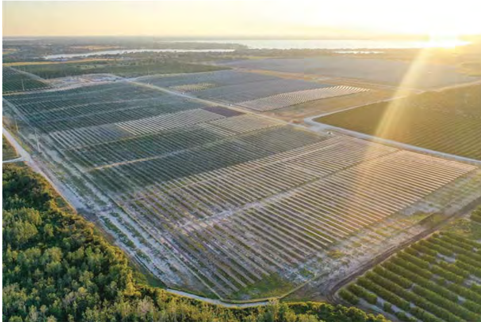
FIGURE 3.6 Lake Placid Solar Site
