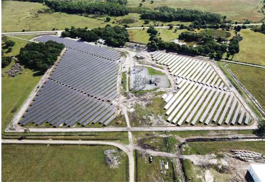
FIGURE 3.2 Osceola Solar Site
