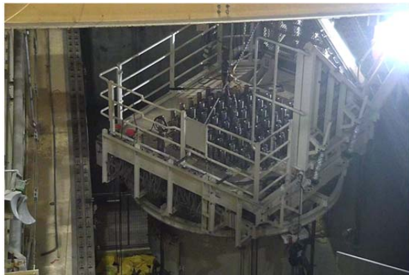
Removal of CRDM Cables
