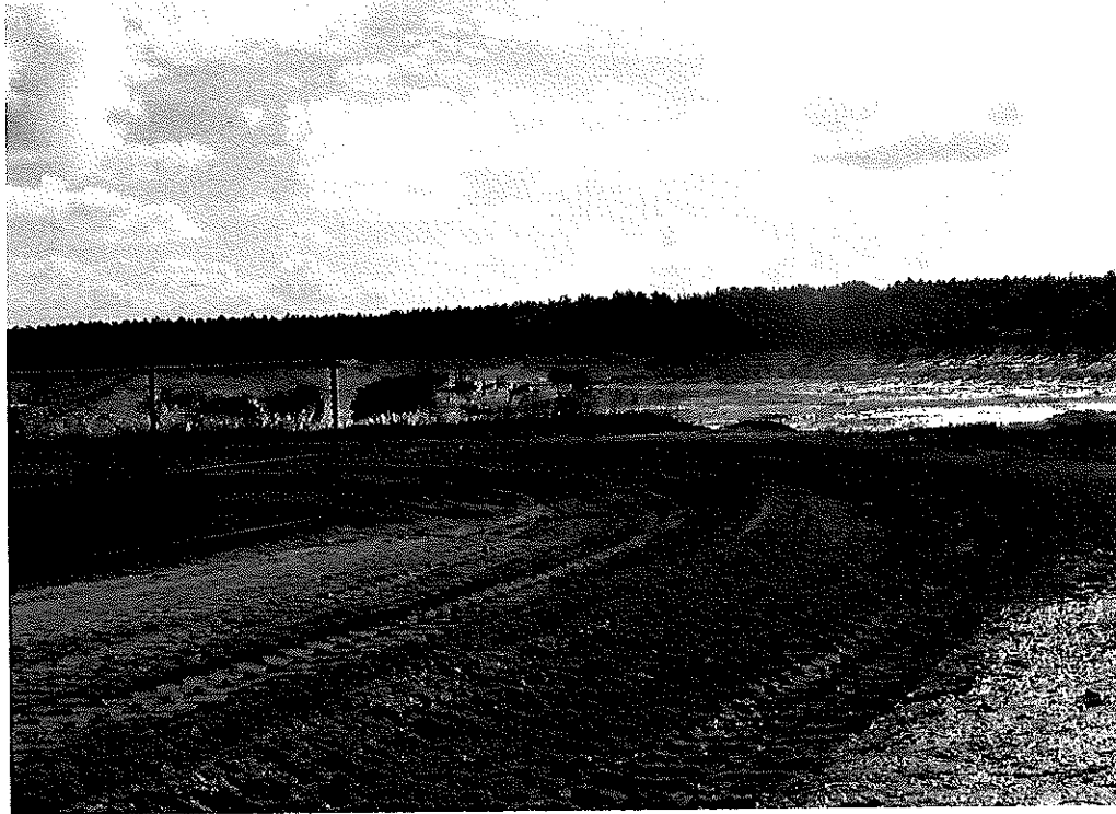
Photograph 5 – View to the southeast showing the outparcel developed as a borrow pit off the south-central portion of the property.
