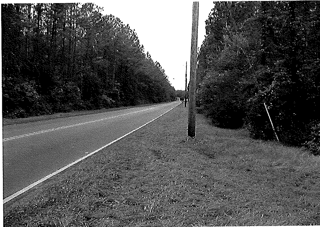
Photograph 12 – View to the west along the Trail Ridge Landfill access road.
