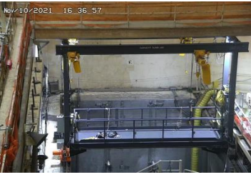
Working Bridge Installed
