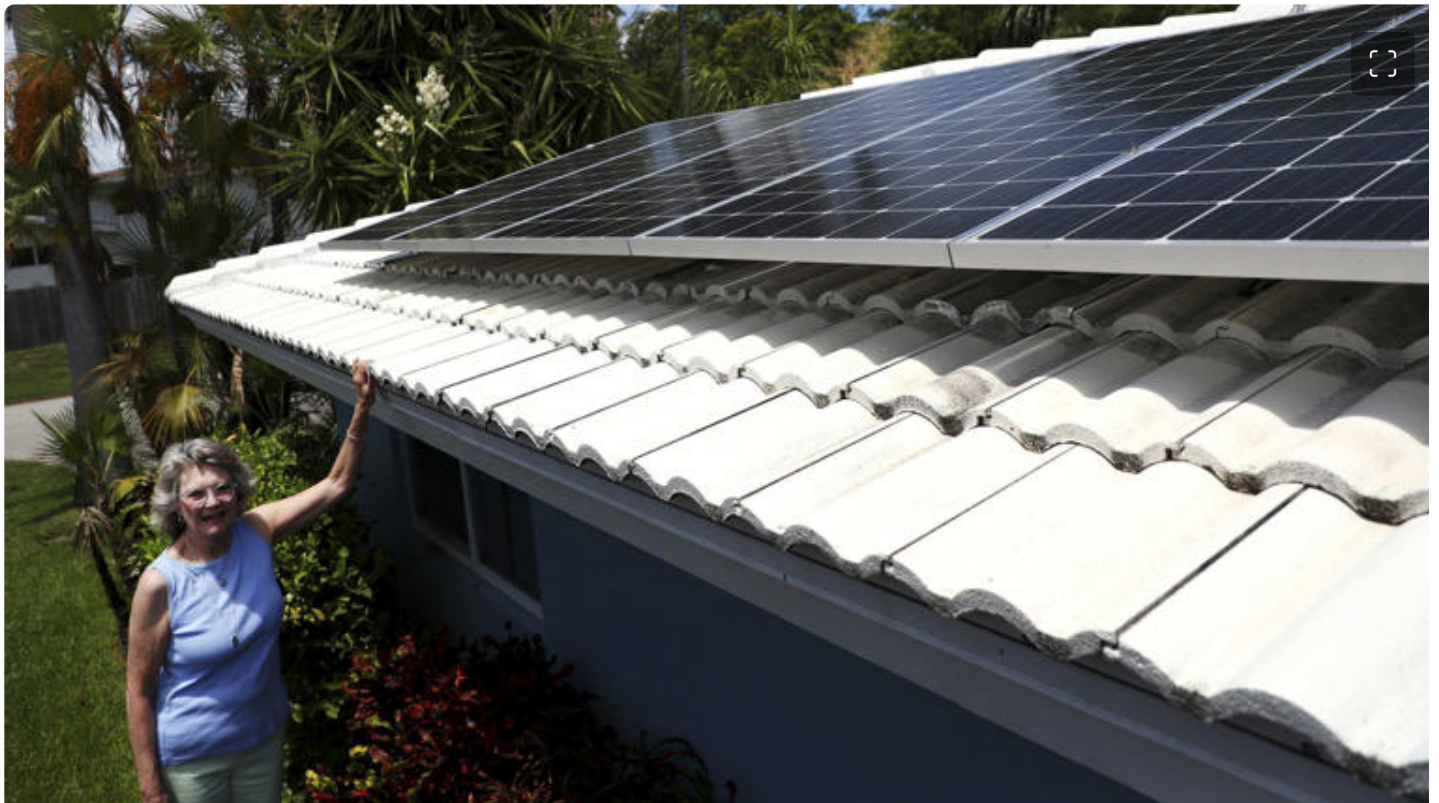
Holly Strawbridge of Oakland Park shows her rooftop solar panels. She's one of an increasing number of solar owners who say their insurers won't cover homes with solar systems.
