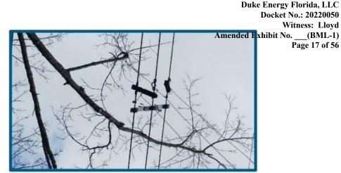
Figure 4: Three examples of open wire secondary that will be addressed
