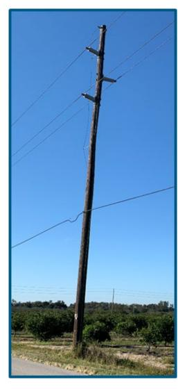
Figure 1: Wood Pole to Non-Wood Upgrade candidate
