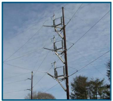
Figure 3: DEF Manually Operated Switch
