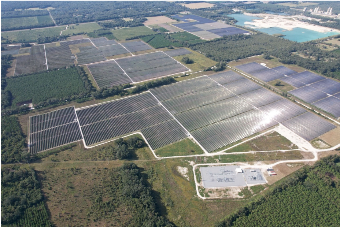
FIGURE 3.5 Hildreth Power Plant
