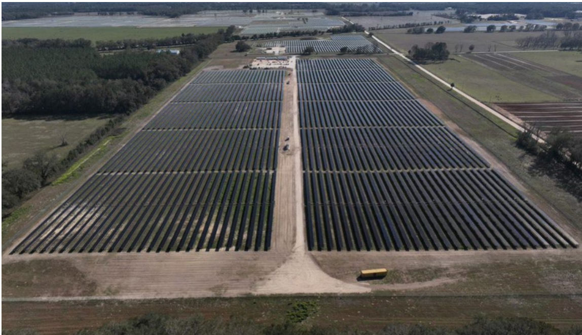
FIGURE 3.3 Hardeetown Solar Power Plant
