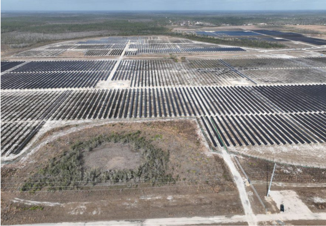
FIGURE 3.2 Bay Ranch Solar Power Plant
