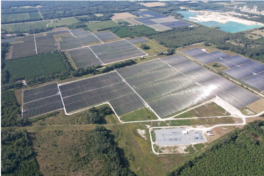
FIGURE 3.5 Hildreth Power Plant
