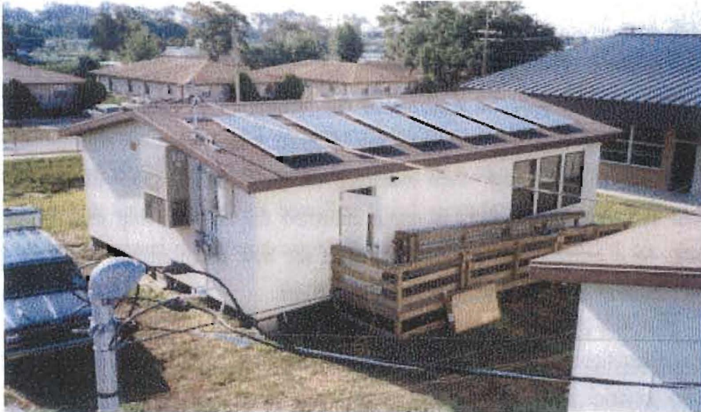
Figure 4-2 Portable Classroom Topped by PV Panels
