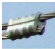
PARALLEL GROOVE (FOR ALUMINUM TO ALUMINUM CONNECTIONS)
