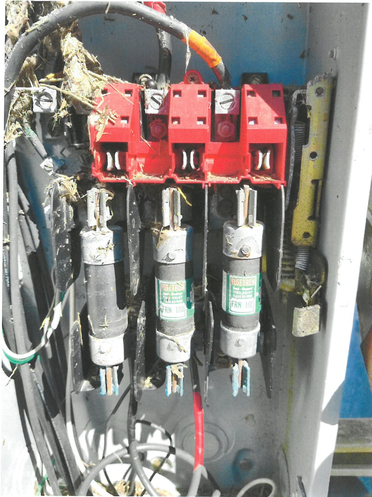
Americus Lift Station Control Panel Flooded by Salt Water Surge (note the seaweed & grass)
