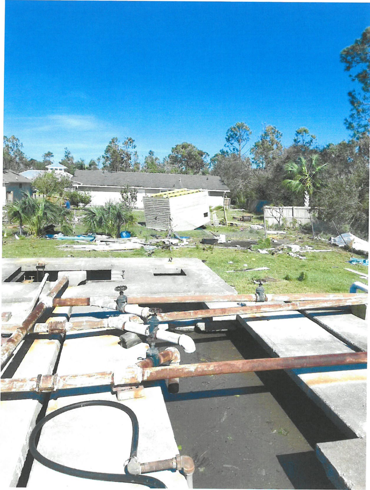
WWTP After Storm Plant Building Overturned & Chain-link Fence Collapsed
