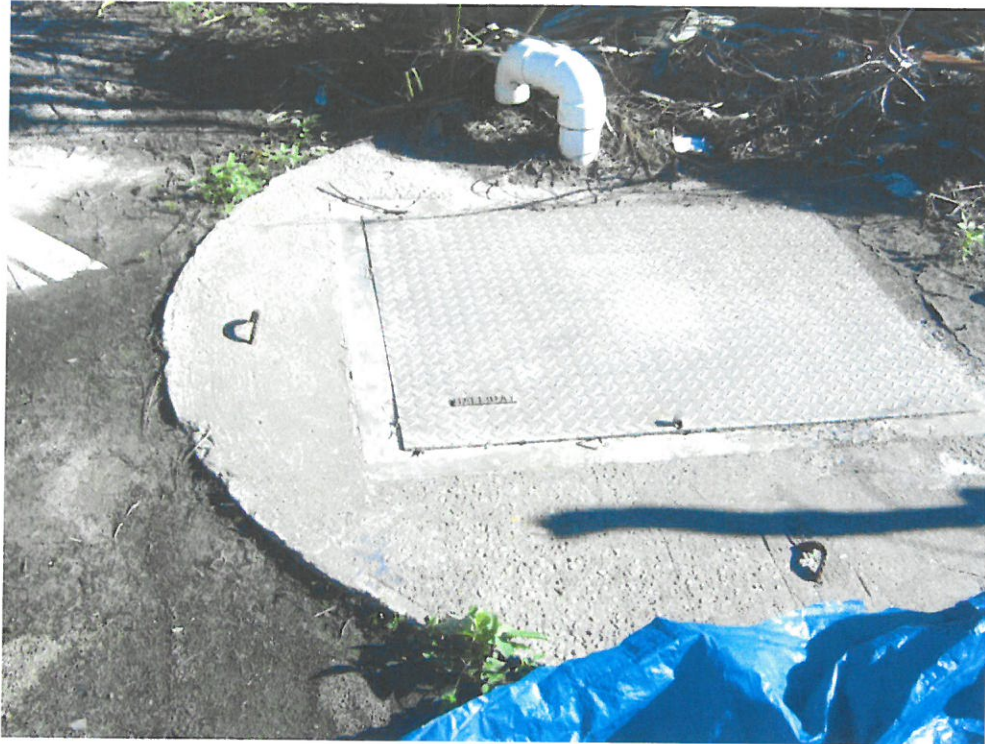
Americus Lift Station After Storm Top needs to be raised
