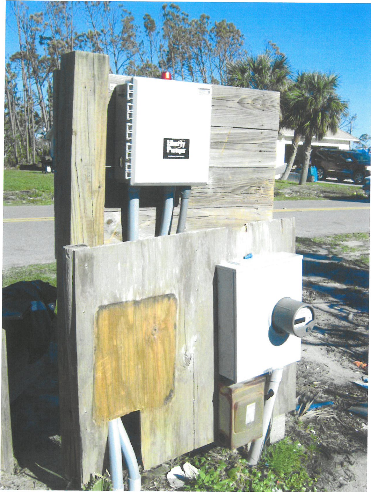
Americus Lift Station After Storm New Control Panel
