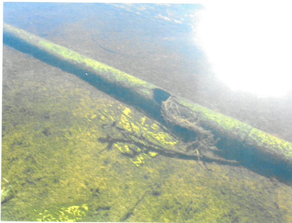
WWTP Polishing & Percolation Pond Piping Damages After Storm
