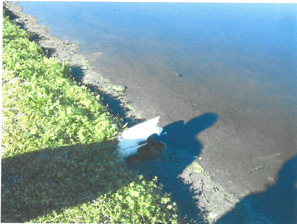
WWTP Polishing & Percolation Pond Piping Damages After Storm
