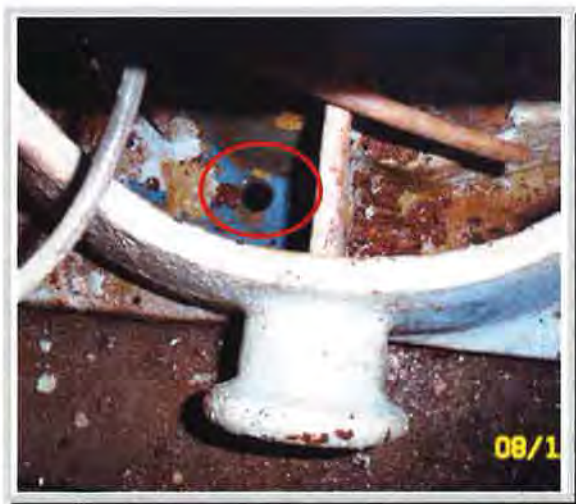
Well 2 at office. Improper well casing vent.
