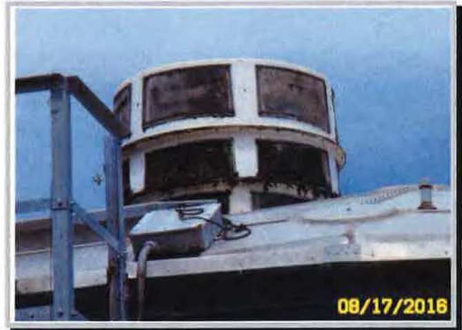
Aerator at Tank 1 Well 2 - 316,000 gal tank.
