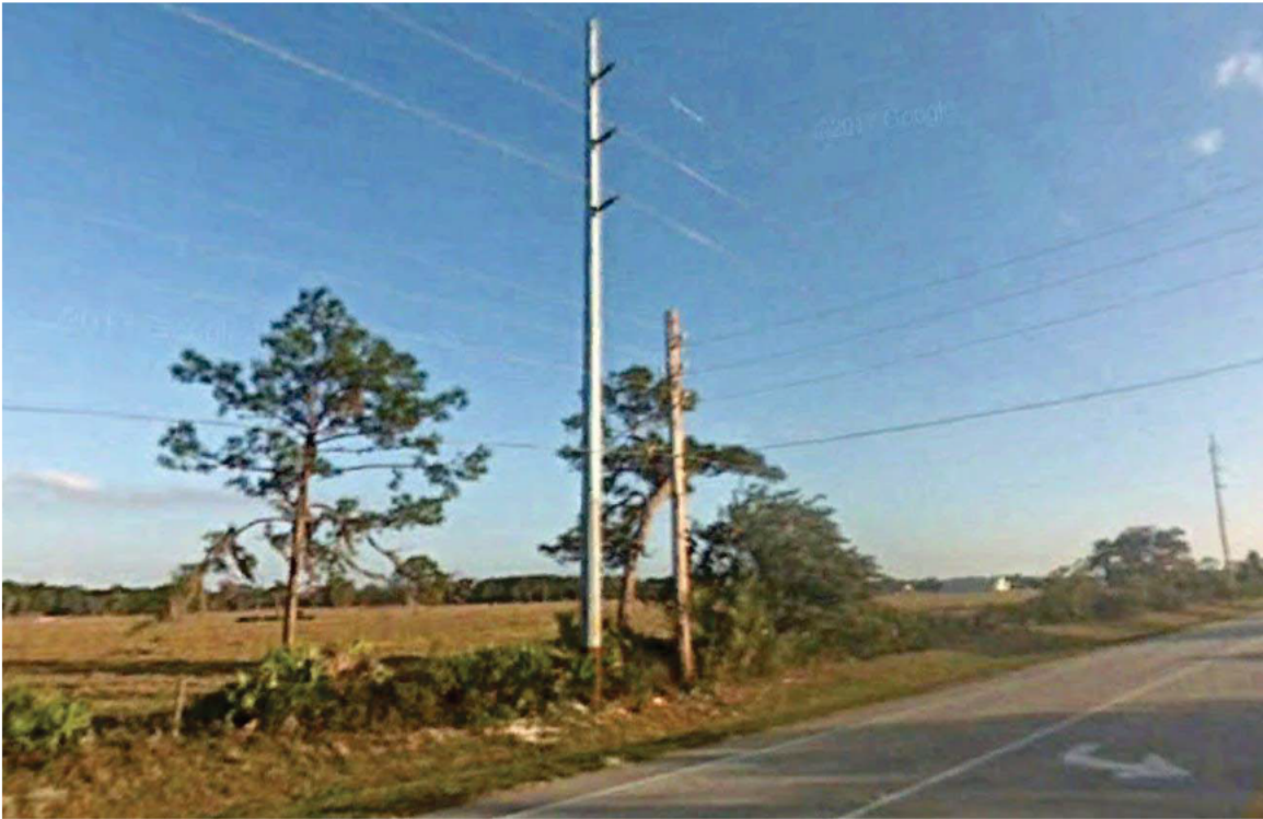
Figure 4: Existing LD steel pole ALP-222 was undamaged and left in place, looking southeast.
