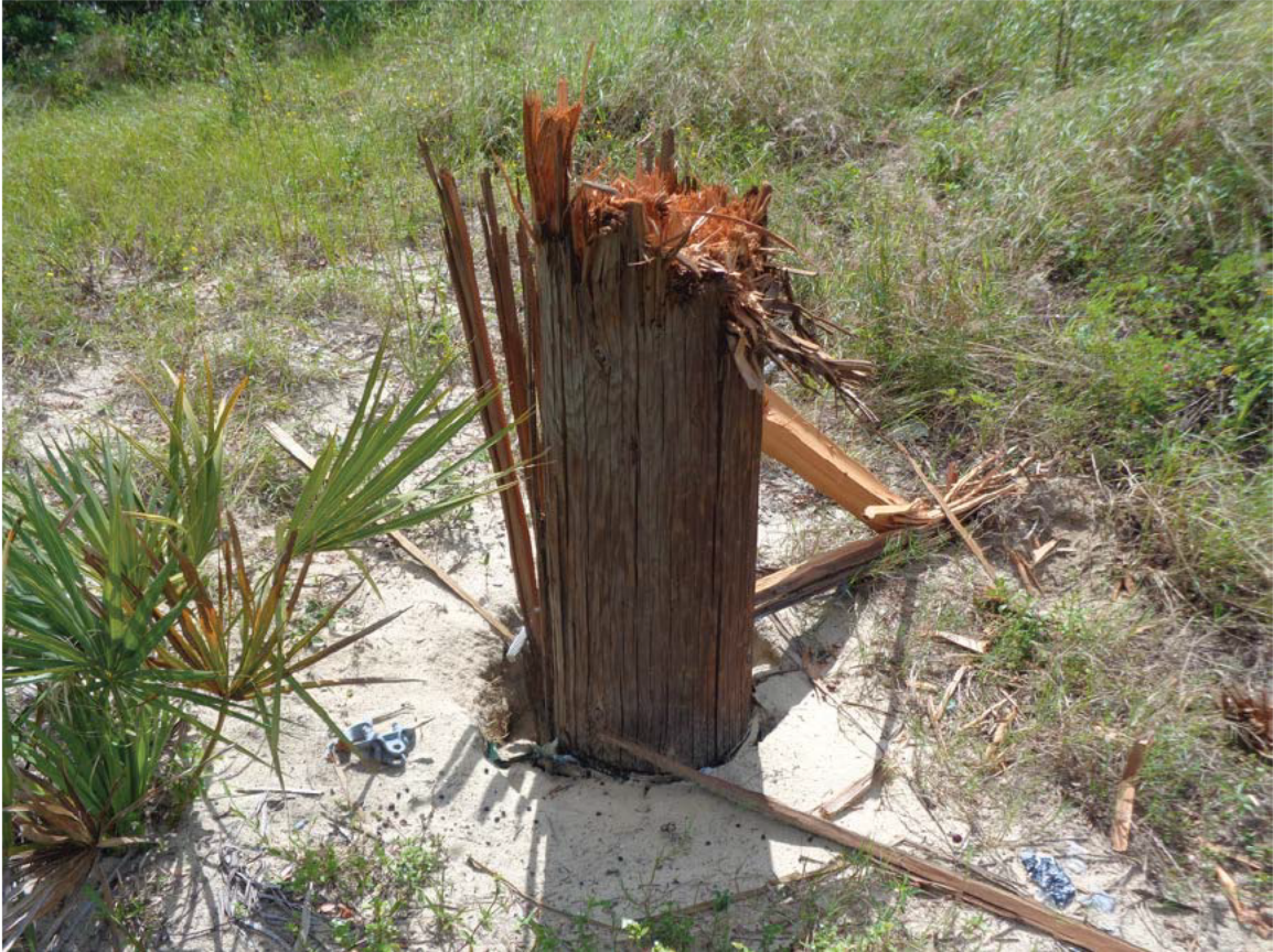
Wood pole AD-16 pole base. Looking southeast.
