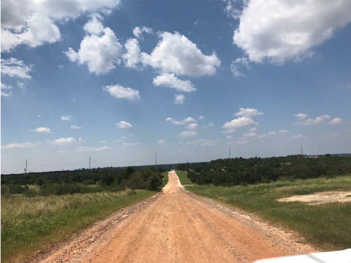
Country Oaks to Dundee 69kV transmission line wind exposure.
