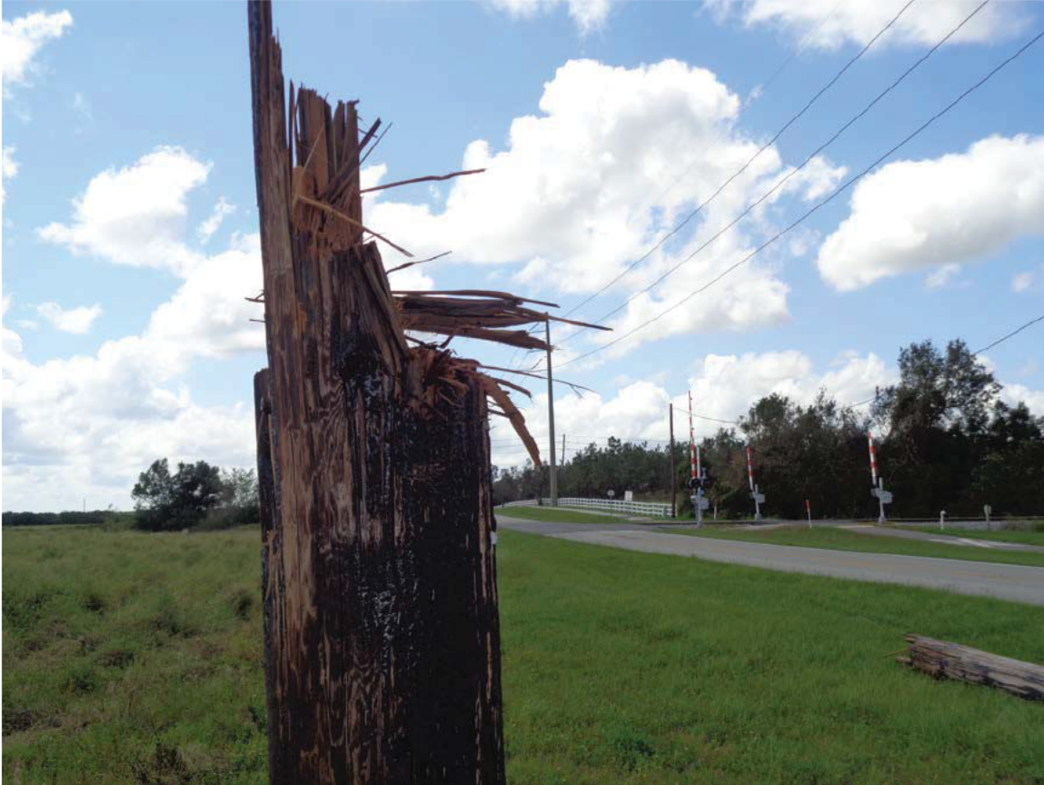
Wood pole AD-14 base. Looking south.
