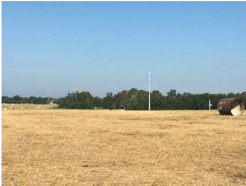
Tower HG-159 replacement.
