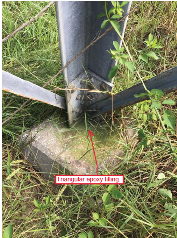
Tower HG-157 epoxy treatment.
