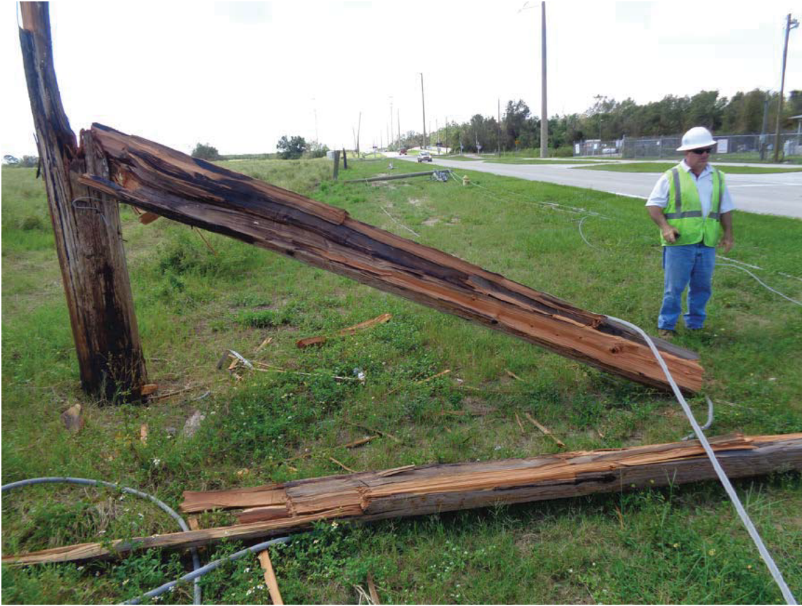
Wood pole AD-13 base. Looking south.
