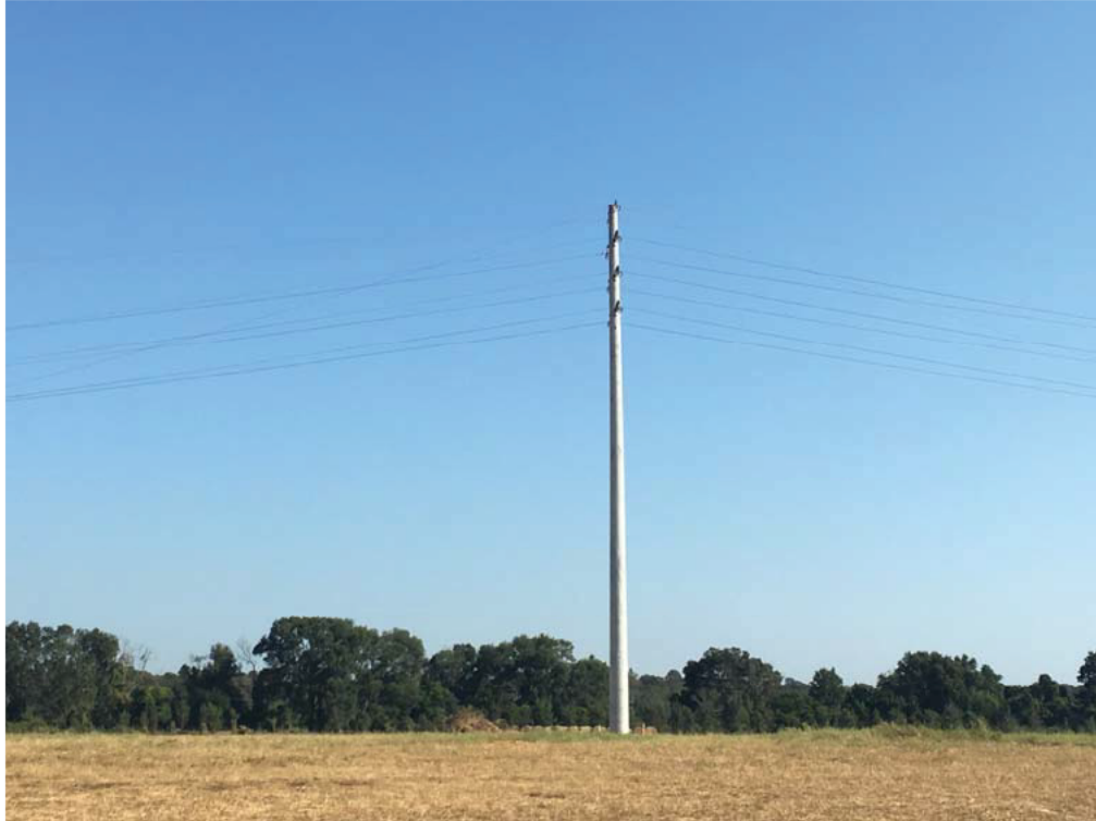
Tower HG-160 replacement.
