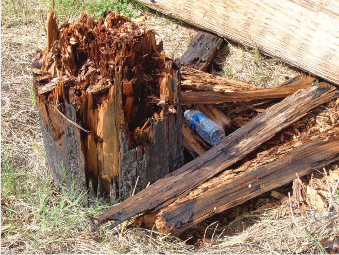
Wood pole AD-20 base. Looking south.
