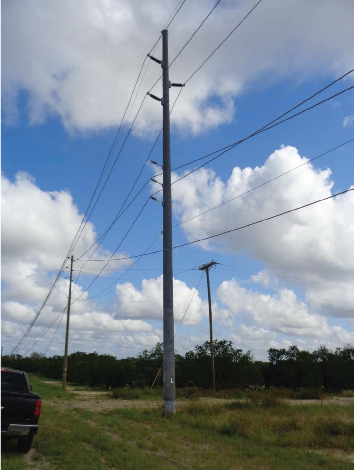
Steel pole AD-23. Looking northeast.
