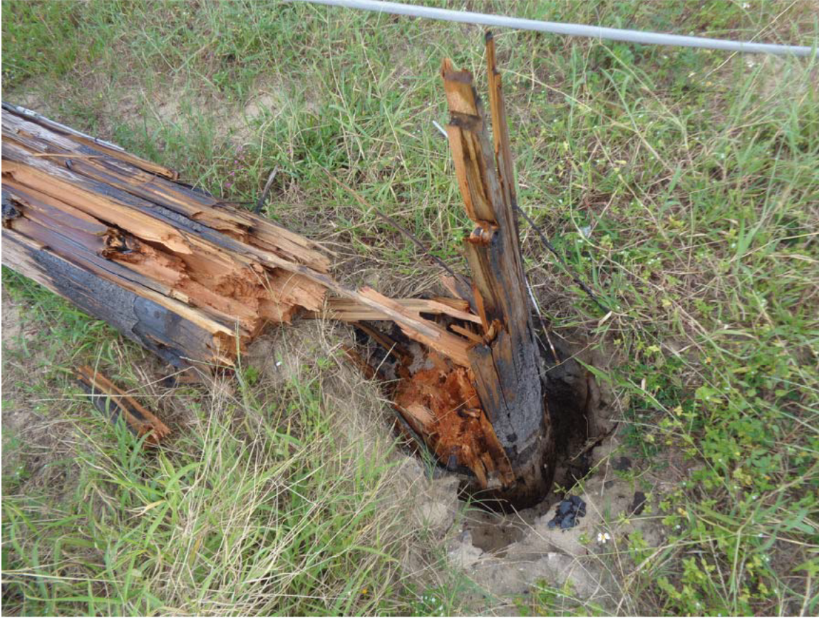
Wood pole AD-18 base. Looking west.
