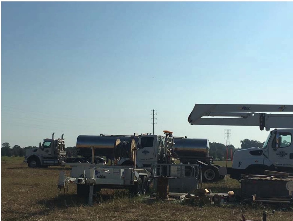
Tower HG-161 replacement.
