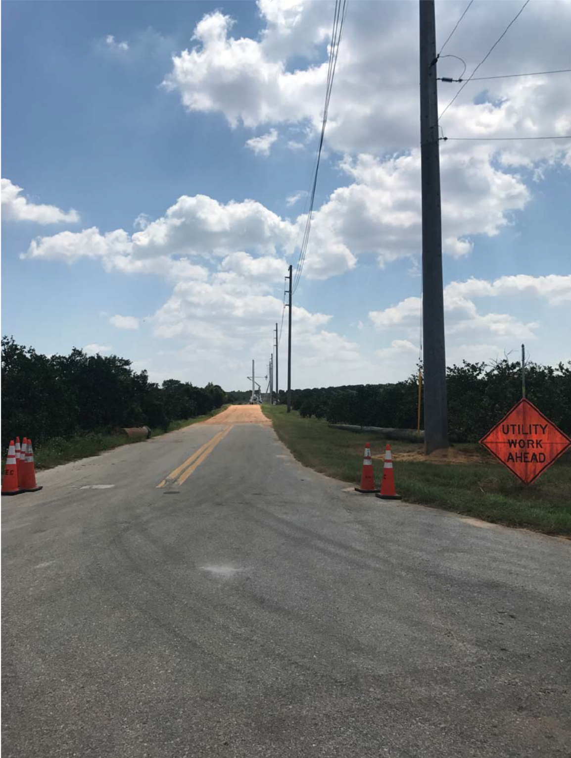
Replaced pole DCO-72. Looking south.
