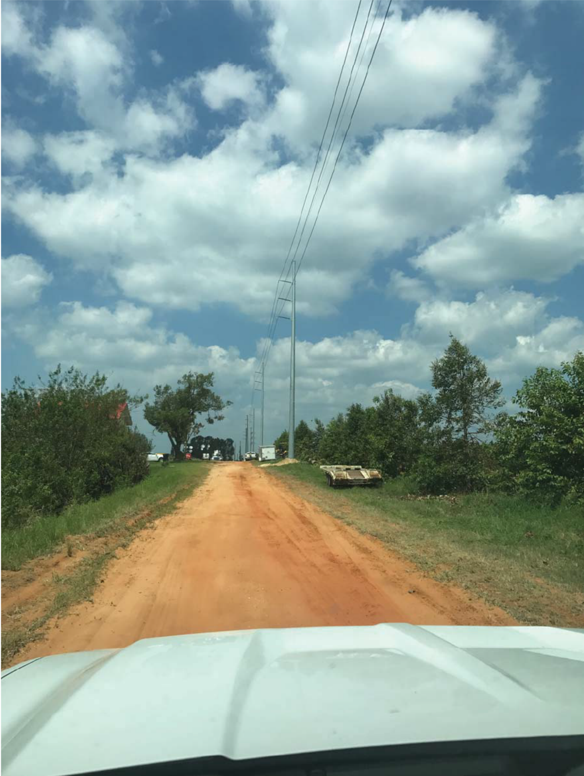
Replaced light duty (LD) steel poles AL-14-5 to AL-14-3. Looking north.
