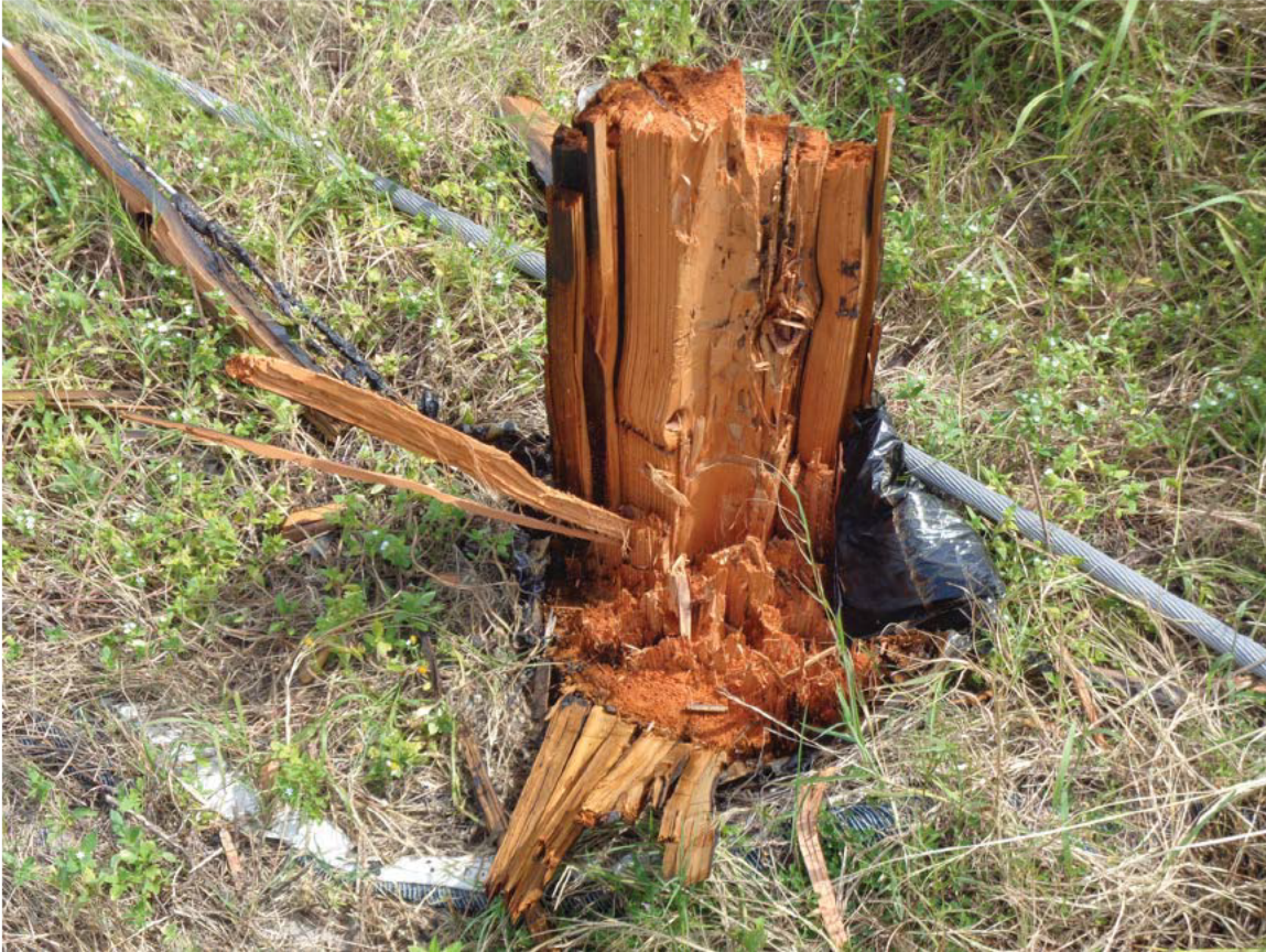
Wood pole AD-19 base. Looking northeast.
