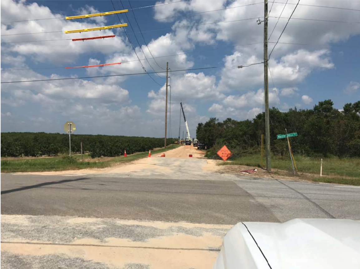
Steel poles DCO-80 to DCO-76 replacement in progress. Looking north.
