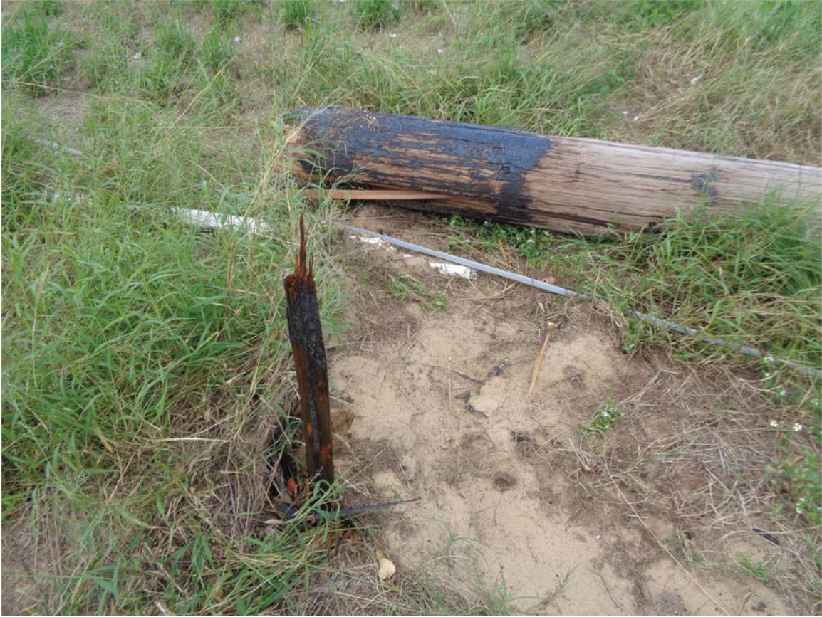
Wood pole AD-22 pole base. Looking west.
