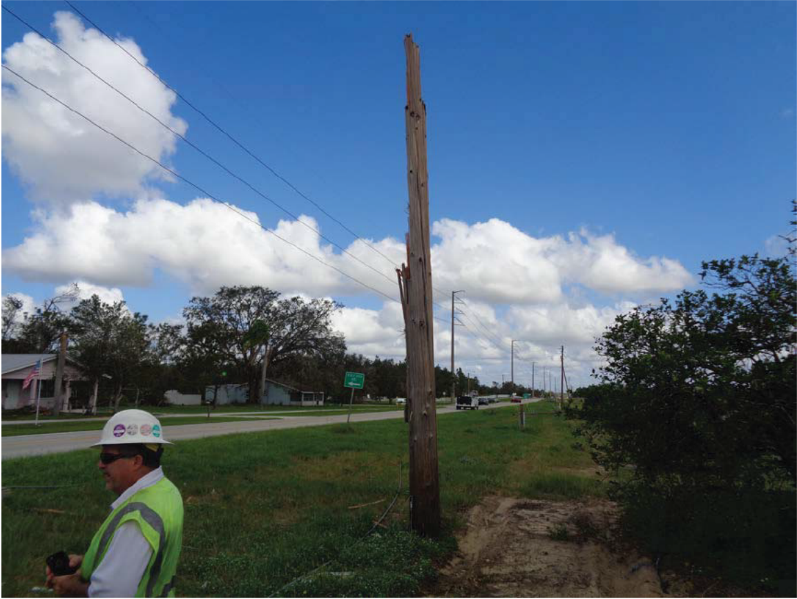
Wood pole AD-21 pole base. Looking southwest.
