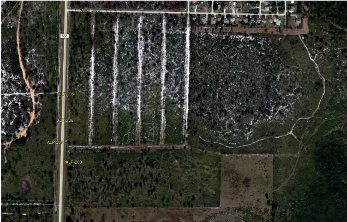
Figure 2: Open area east of transmission line exposed structures to westbound hurricane winds.
