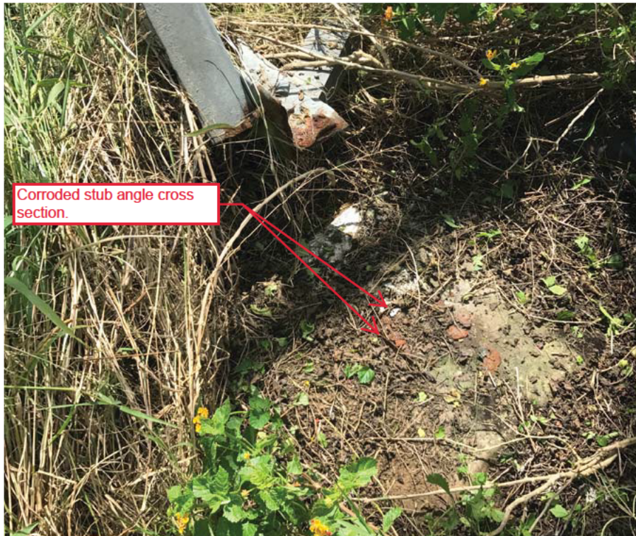
HG-160 SE foundation, corroded-sheared stub angle.
