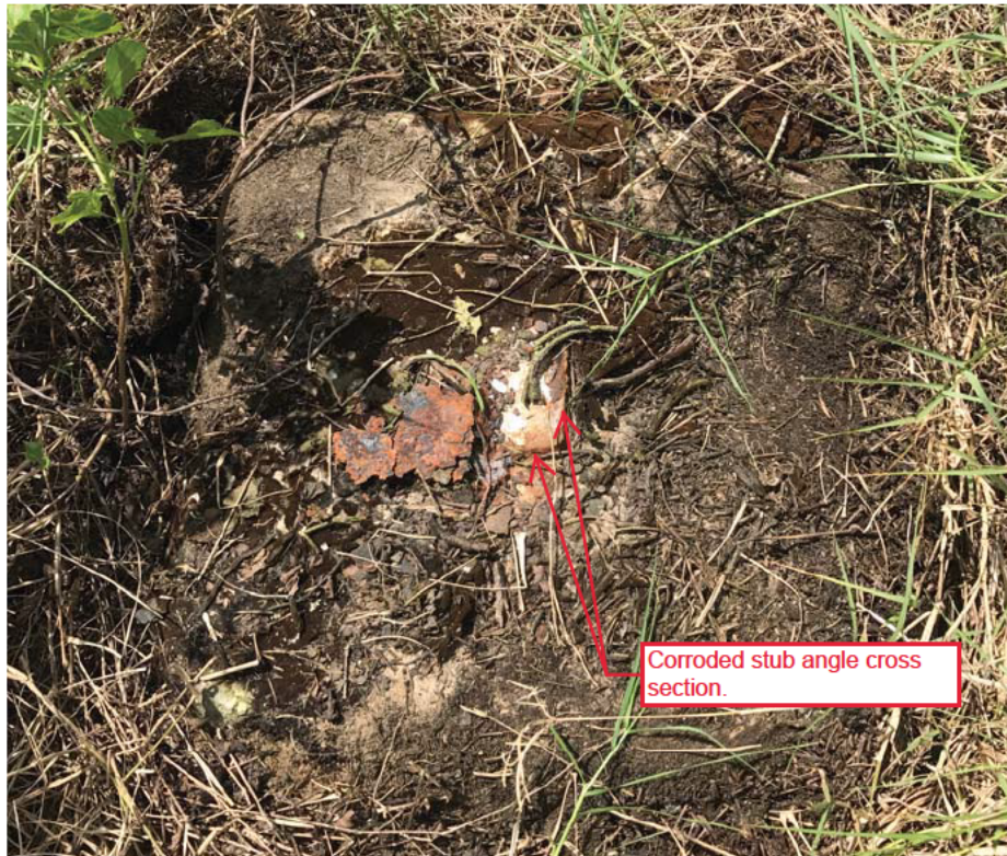
HG-160 NE foundation, corroded-sheared stub angle.
