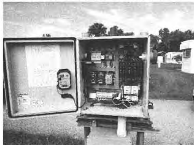
18. Electrical panel for lift station
