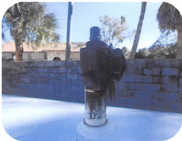
7. Pressure Release Valve Missing Tag
