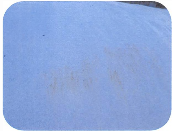
6. Coating Failure with Surface Corrosion
