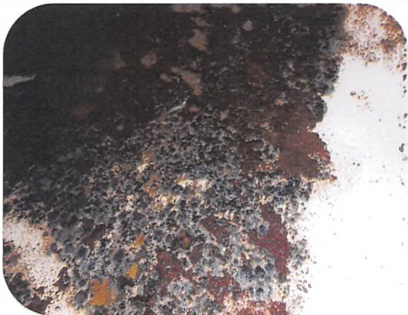
15. Internal Coating Failure on Lower Shell
