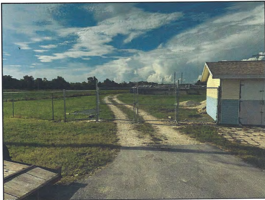
PHOTO 5 NEW PLANT ACCESS GATE
