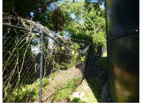
Photo 14: View of broken fence.
