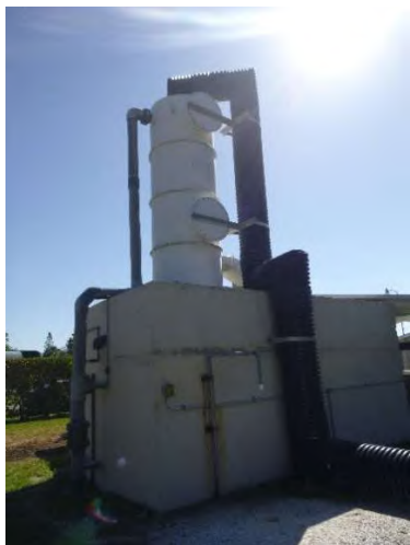
Photo 5: View of Forced Draft Aerator.
