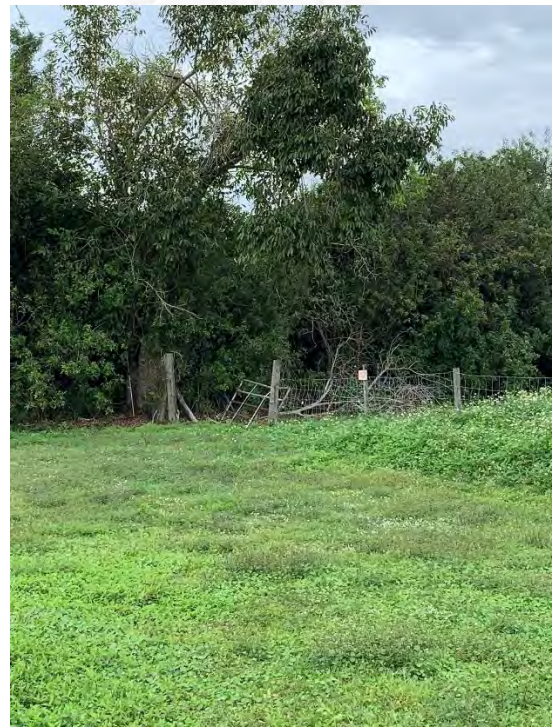
30. Broken Gate on Disposal Site Fence
