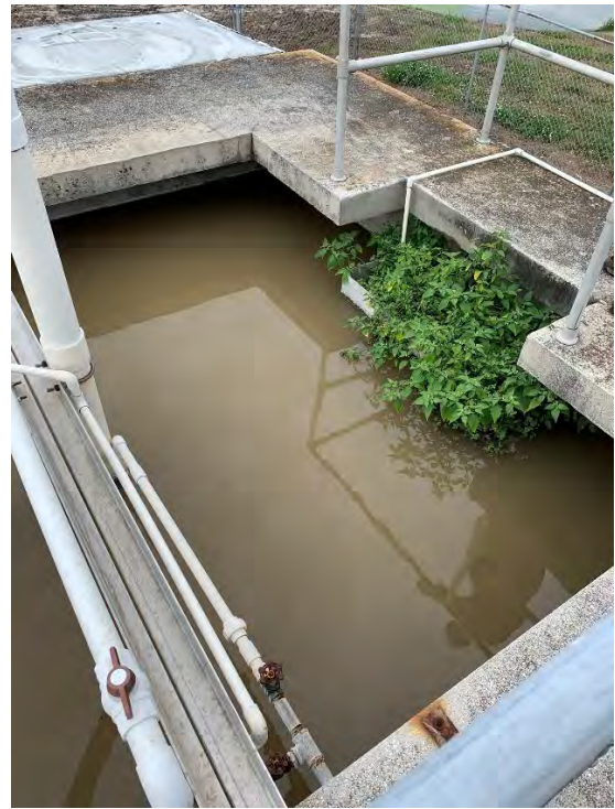
18. Stilling Well with Vegetation
