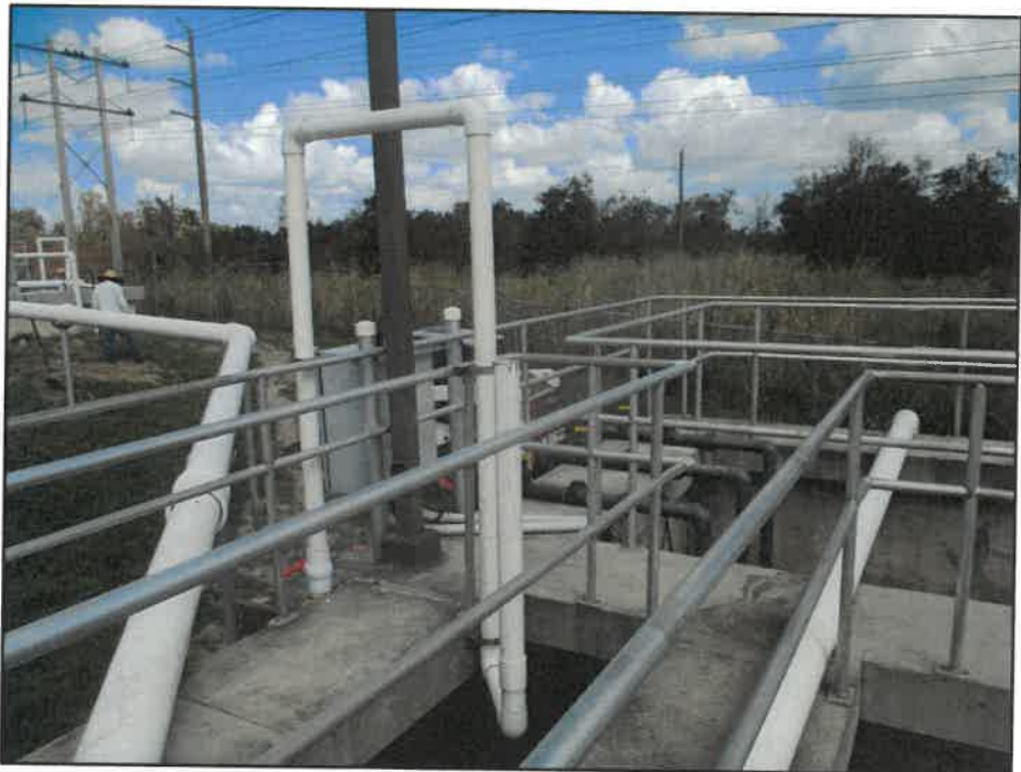
PHOTO 12: WAS PIPING TO SOUTH DIGESTER
