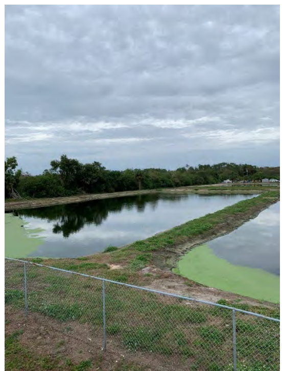
24. Rapid Infiltration Basin
