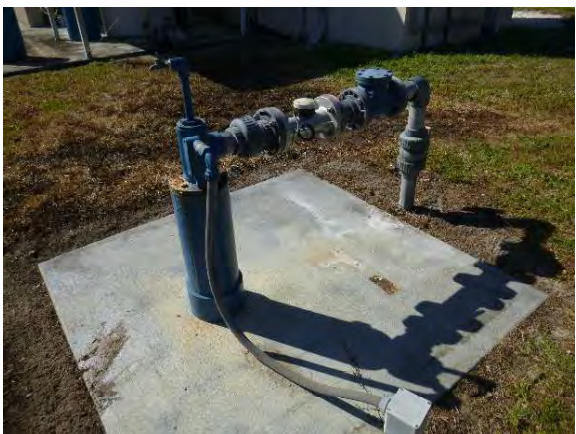
Photo 3: View of Well.
