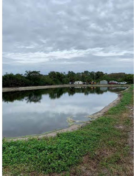
26. Rapid Infiltration Basin
