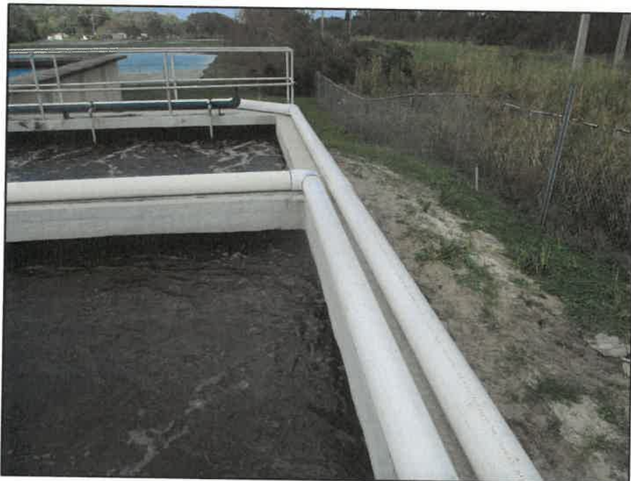
PHOTO 8: INFLUENT PIPING SUPPORTED ON TOP OF TANK WALLS
