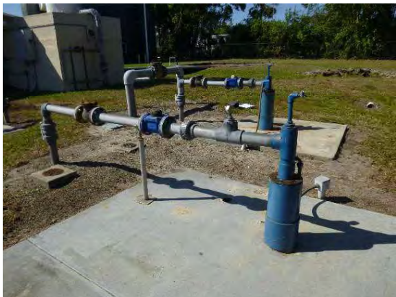
Photo 1: View of Well.
