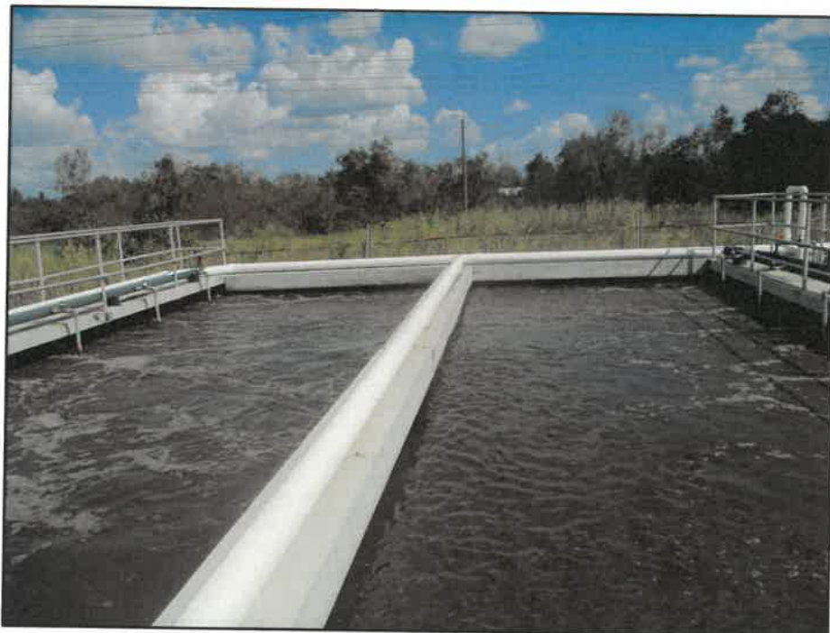
PHOTO 6: PROCESS PIPING SUPPORTED ON TANK TOP OF WALL SOUTH PLANT
