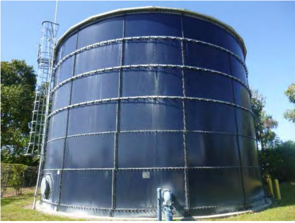
Photo 13: View of Ground Storage Tank.
