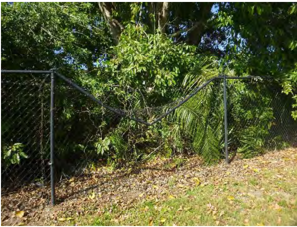
Photo 15: Continued view of broken fence.
