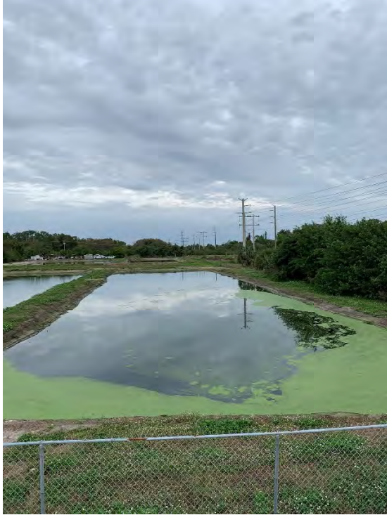
25. Rapid Infiltration Basin
