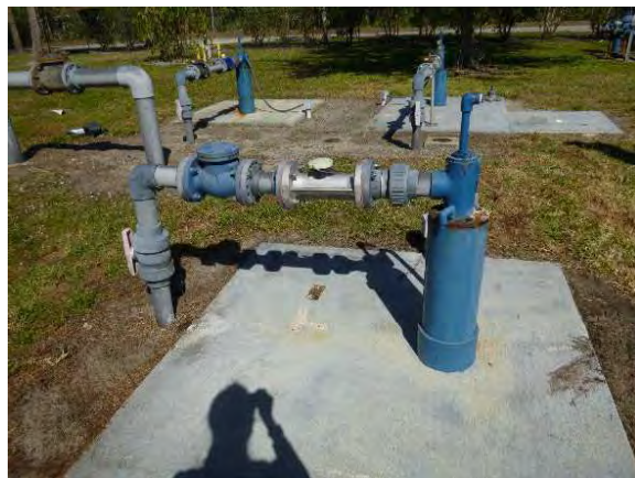
Photo 4: View of Well.
