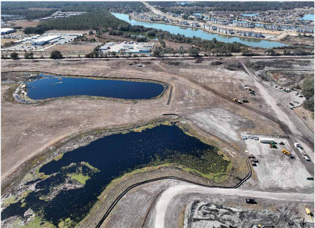
Figure 7-6: Edge Solar - Project Site under construction
