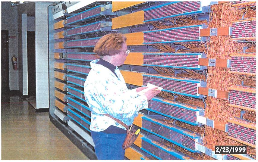
Step 8: Technician locates and removes end of jumper connected to the BellSouth cable pair.
