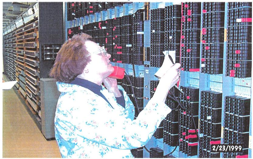
Docket Number 990750-TP Step 6: Technician walks along Main Distributing Frame to locate both ends of jumper to be cut.
