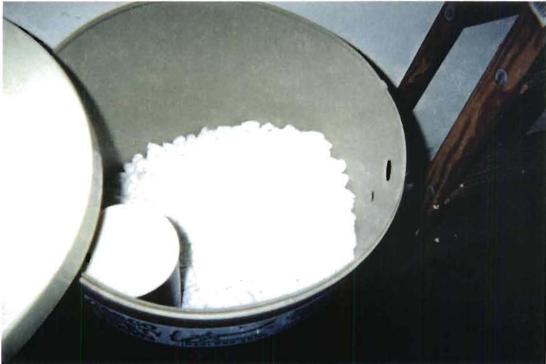
WATER SOFTENING SALT PELLETS AT COOGAN RESIDENCE
