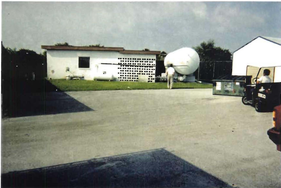
YARD VIEW OF WELL NO. 1
