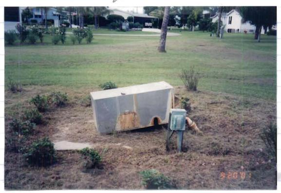
This wew shows disrepair of ancillary equipment. Cover is not secured. Weighbors keep weeds cut & have planted shrubs around area to try & hide an eyerore in their backyards.
