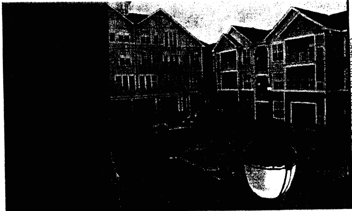
Brentmoor Apartments in Raleigh, North Carolina
