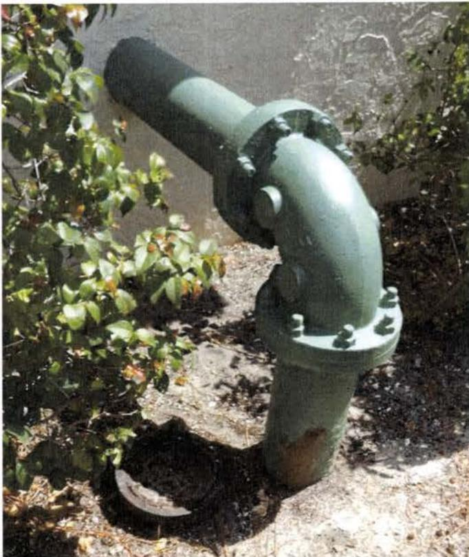
Figure 3. Corrosion observed on pipe leading from pump house for well#1.
