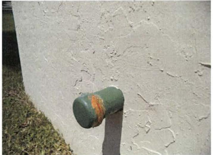
Figure 8. Corrosion on flush-line cap at well#3.
