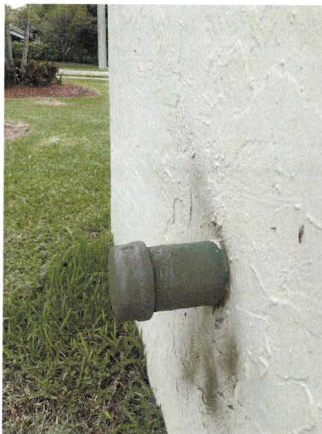
FIGURE 8. WELL #3 FLUSH LINE CAP TIGHTENED, WIIRE BRUSHED, AND ANTI CORROSION COATED.
