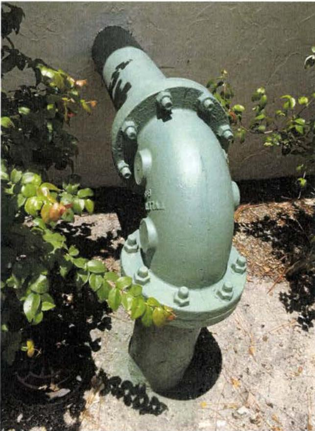
FIGURE 3. CORROSION ON WELL #1 DISCHARGE PIPE WIRE BRUSHED, ANTI CORROSION COATED.
