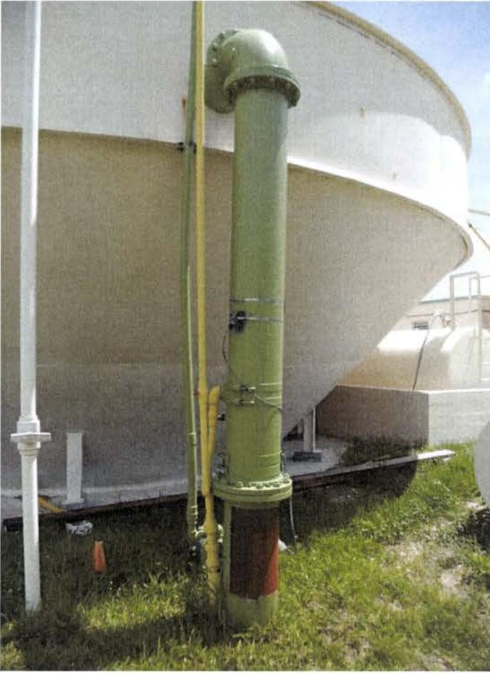
Figure 9. Corrosion on manifold pipe leading to Accelerator.
