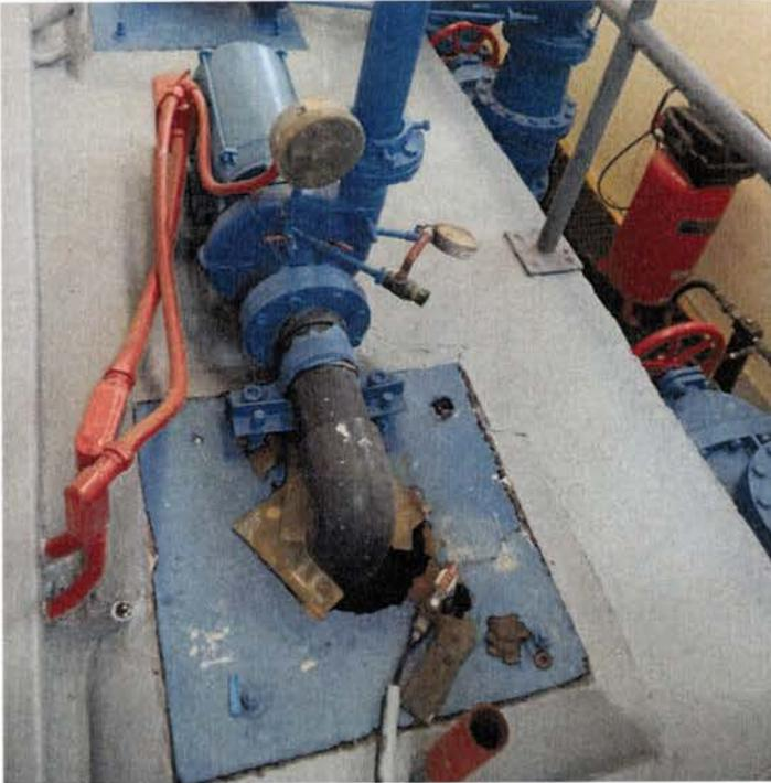
Figure 1. Hole observed in top of the clearwell.
