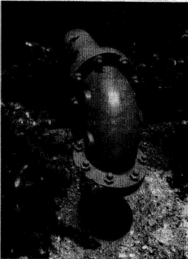
**FIGURE 3. CORROSION ON WELL #1 DISCHARGE PIPE WIRE
