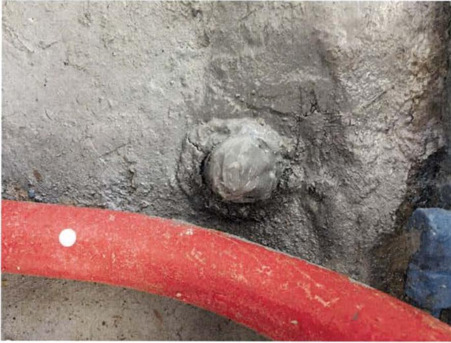
FIGURE 13. HS PUMP #2 DEAD WIRES IN ABANDONED CONDUIT SEALED & COATED.
