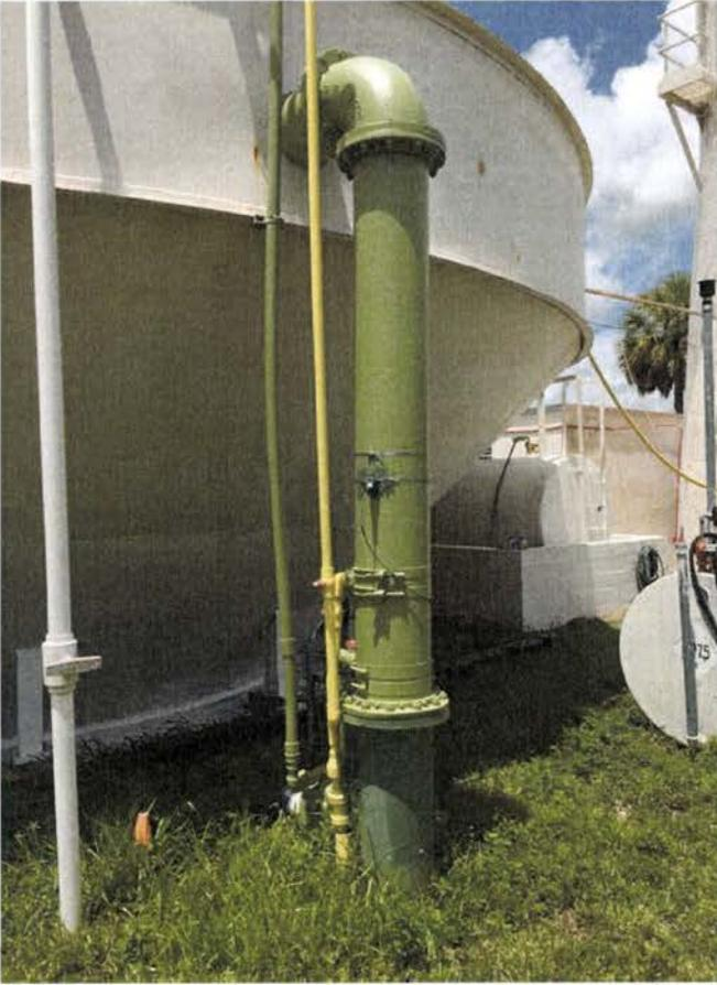
FIGURE 9. RAW WATER RISER METER TEST AREA WIRE BRUSHED AND ANTI CORROSION COATED.
