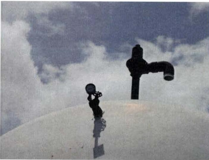
Figure 15. New pressure gauge installed on hydro tank.
