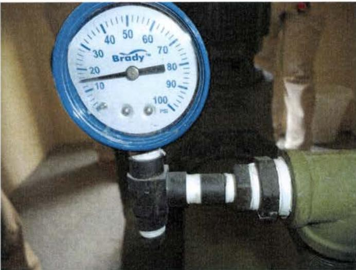
Figure 5. Broken pressure gauge at well#2 (corrected on site, see figure 6).
