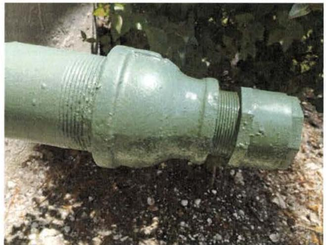
FIGURE 4. CORROSION ON FLUSH-LINE WELL #1. FITTING TIGHTENED, WIRE BRUSHED, ANTI CORROSION COATED.
