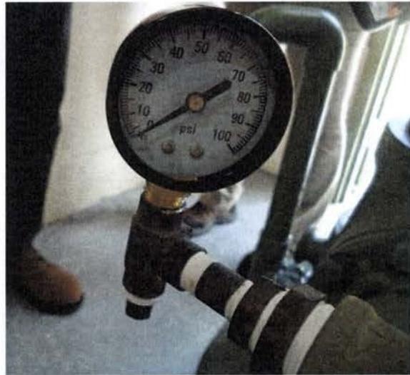
Figure 6. New pressure gauge installed at well#2.
