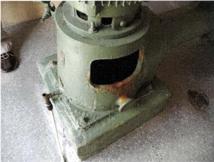
Figure 7. Corrosion observed at the head of well#3.
