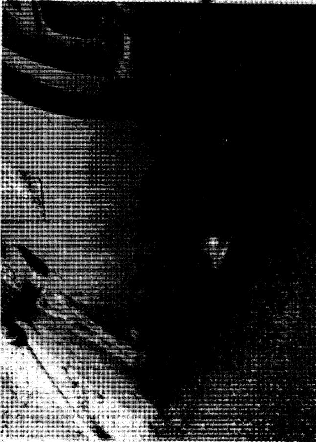
**FIGURE 5. WELL #3 CORROSION AREAS WIRE BRUSHED,
