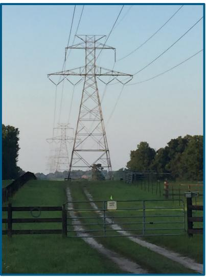
Figure 2: Double Circuit Tower
