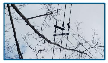
Figure 4: Three examples of open wire secondary that will be addressed
