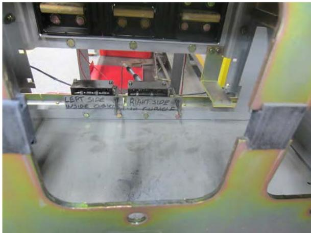
Cell Switches shown through Breaker Rear Panel
