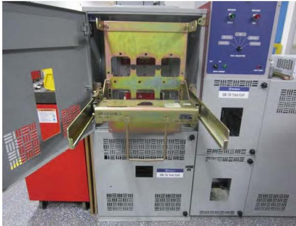
Breaker Frame on Test Cell Rails
