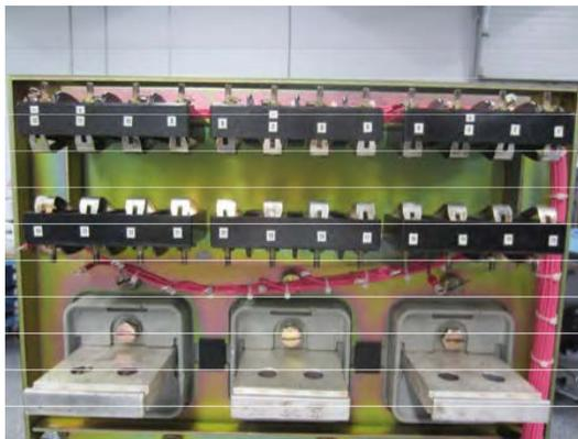
Secondary Contact Assembly on Breaker
