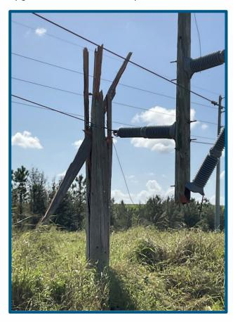
Figure 1: Broken Pole due to extreme weather event.
