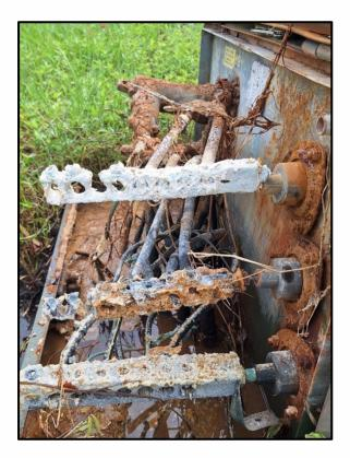
Figure 1: Underground construction with severe corrosion and electrolysis due to storm surge during Hurricane Helene
