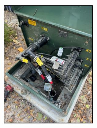
Figure 2: Underground construction with sealed connectors mitigating impacts of storm surge.
