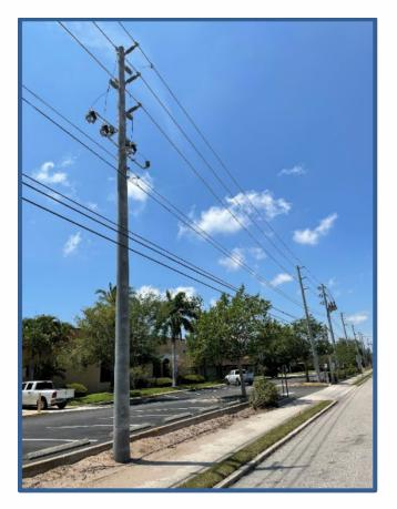
Figure 2: Hardened distribution feeder including structures that have been strengthened to the NESC 250C standard and increased BIL from hardware and spacing upgrades.
