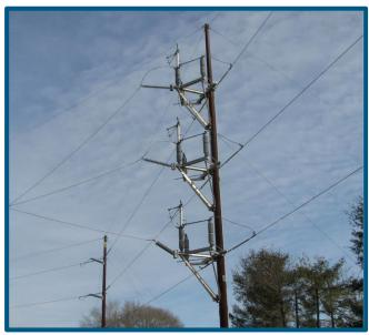
Figure 5: DEF Manually Operated Switch
