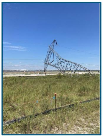
Figure 4: Lattice Tower impacted by Hurricane Idalia
