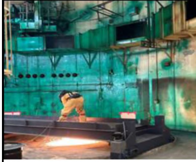
RB 95 Downsizing bridge in Bravo D-Ring
