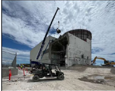
Raised Brokk to Control Complex Roof
