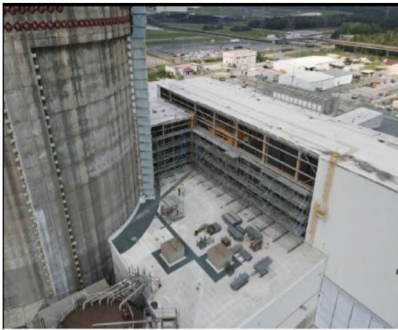
AB Galbestos Siding Removal
