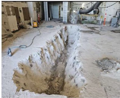
IB 119 Drain Removal Decon
