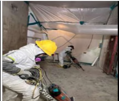
AB 95 Epoxy removal Decon
