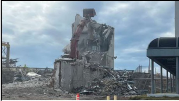
PAB Elevator Shaft Demo
