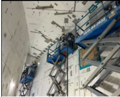
IB 95 Paint Removal Decon
