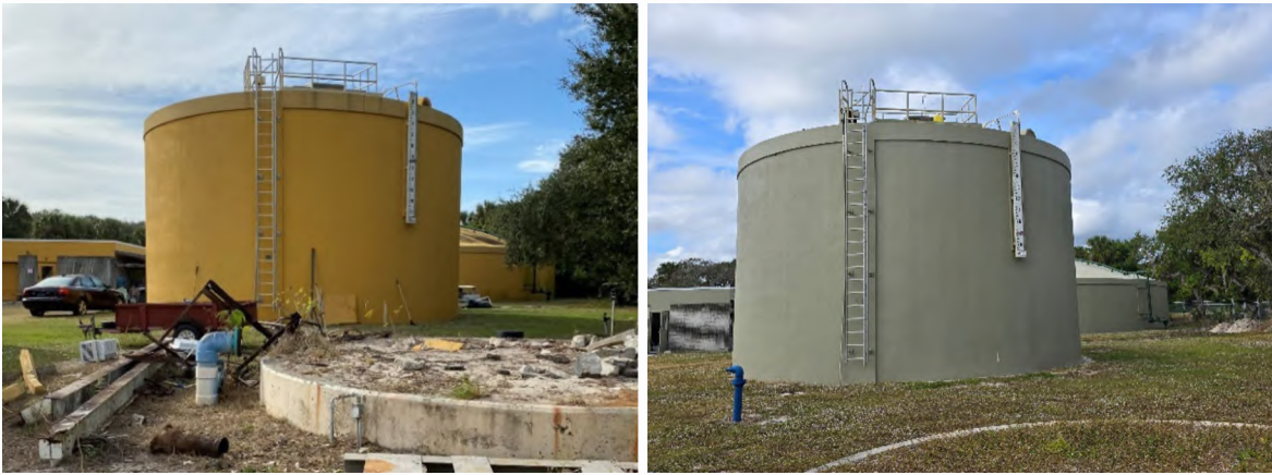
8 9 Ground Storage tank before (left) and after (right) before and after inspection and recoating, 10 note trash and debris removed from tank area as well.
