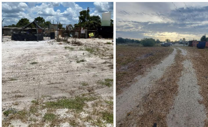
Typical degraded condition of roads and surfaces at acquisition.
