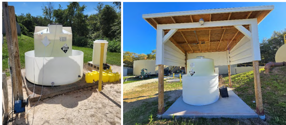
Chemical storage before (left) and after (right) improvement.
