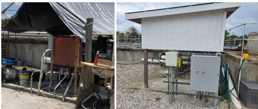
Blower control panel and shade structure before (left) and after (right) improvements, note general cleanup of area from trash and debris as well.
