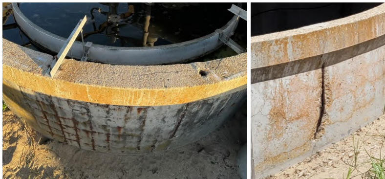
Examples of cracking and exposed rebar in concrete tanks.
