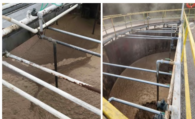
Examples of Aeration headers and drop pipes before and after replacement.
