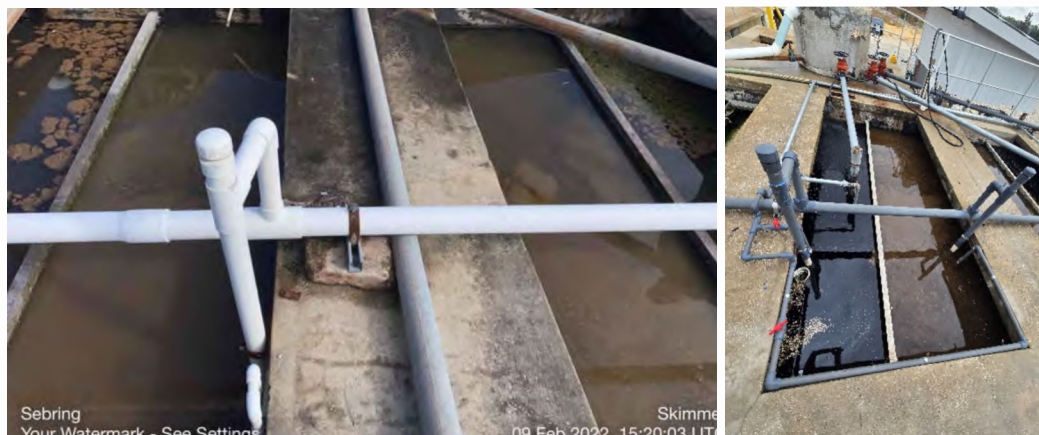
13 14 Old skimmer and air l.f.ts (left) and newly installed air l.f.ts and sludge returns (right), note
