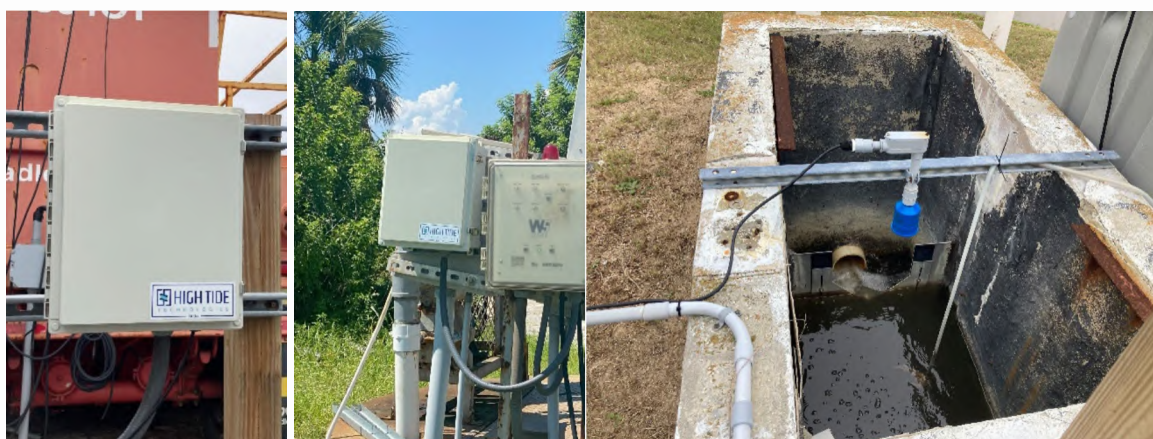
New remote monitoring units installed at the treatment plant (left) and lift stations (center).
