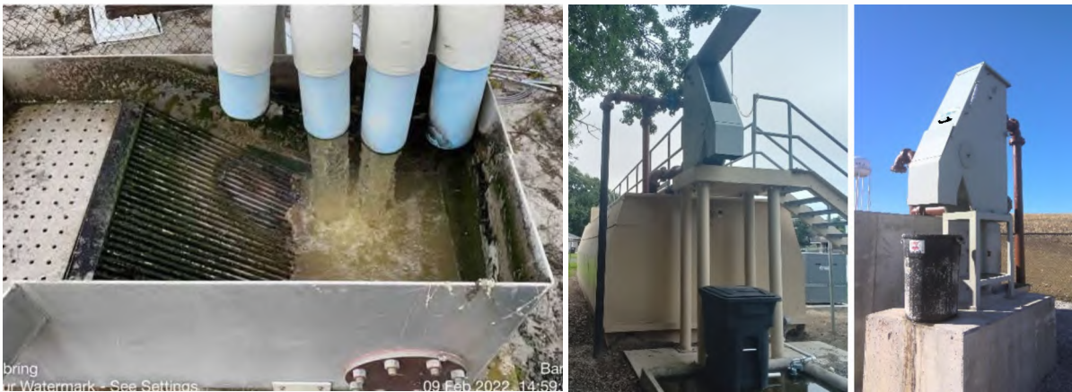
Existing bar screen (left), examples of Hydrosieve with automatic trash collection beneath at two CSWR affiliated facilities (center and right).
