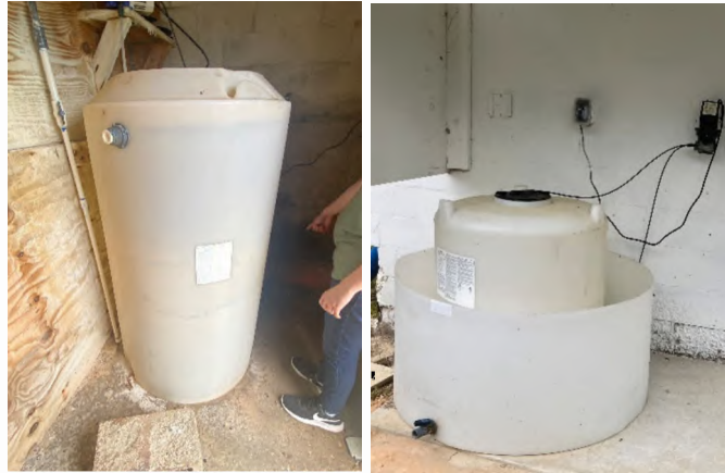
Chlorine storage before (left) and after (right) installation of spill containment.
