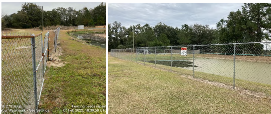
Example of damaged (left) and repaired (right) fencing at the Landfair treatment facility.
