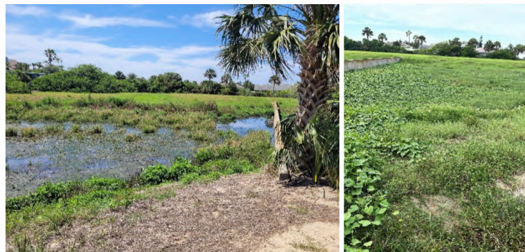
Examples of overgrowth of rapid infiltration basins.
