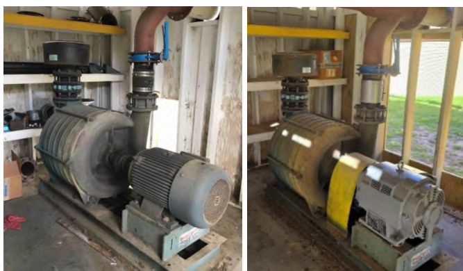
Blower motor before (left) and after (right) replacement, also repair work to blower building underway at time of photo.
