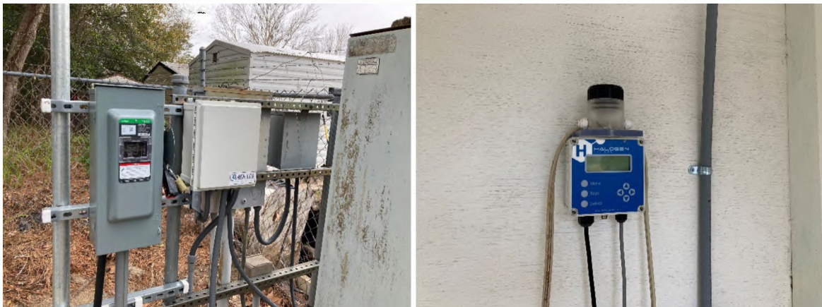
New remote monitoring equipment (left) and new chlorine residual monitoring (right)
