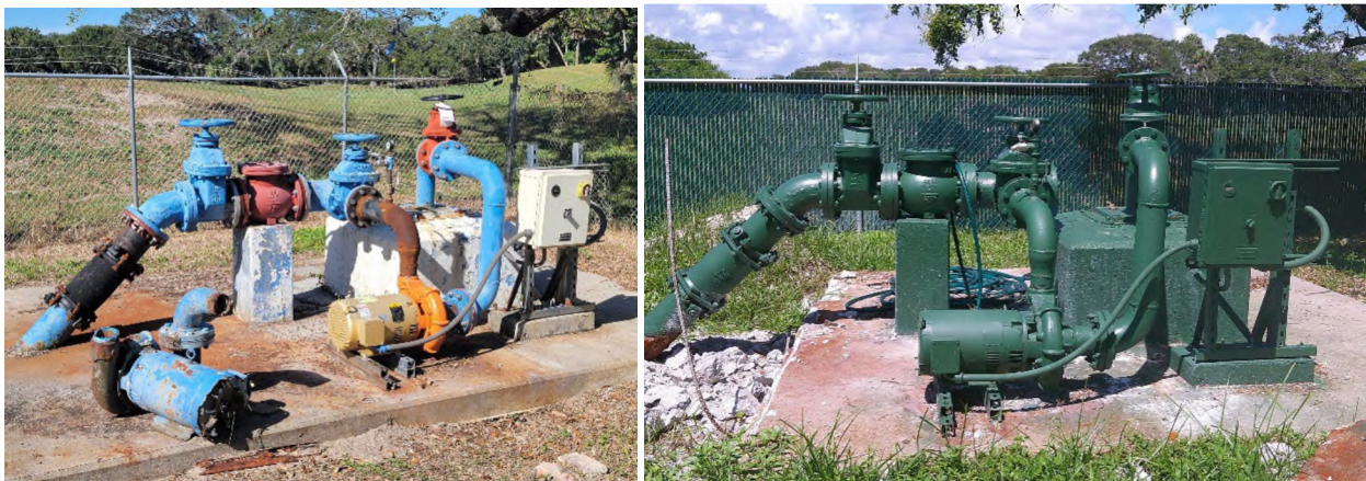
Example of before (left) and after (right) recoating of above ground piping and equipment.
