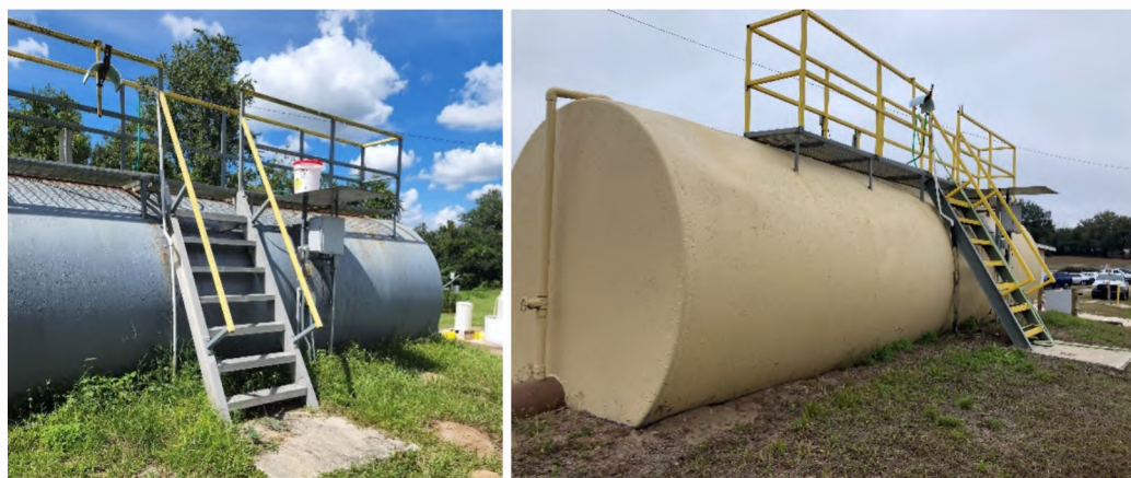
Disinfection mixing tank before (left) and after (right) recoating and repainting handrails
