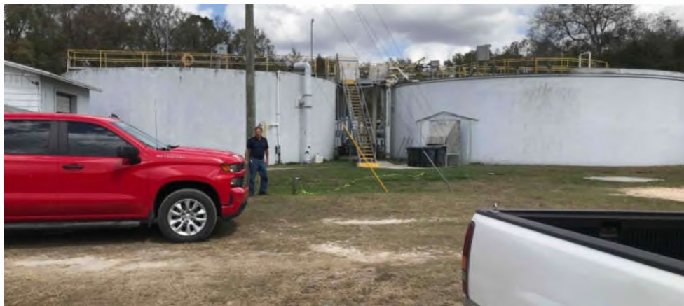
Beverly Hills/Rolling Oaks Wastewater Treatment Facility
