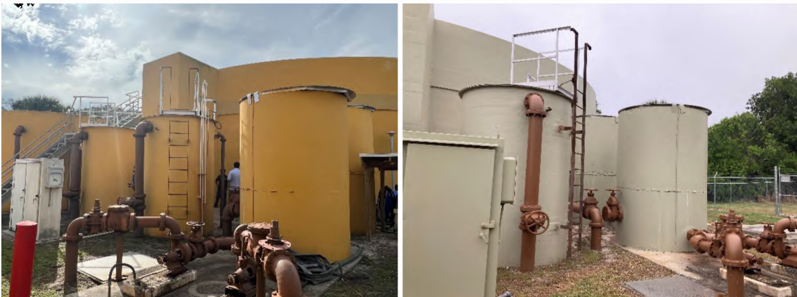
13 14 Treatment tanks, piping, and equipment before (left) and after (right) recoating.
