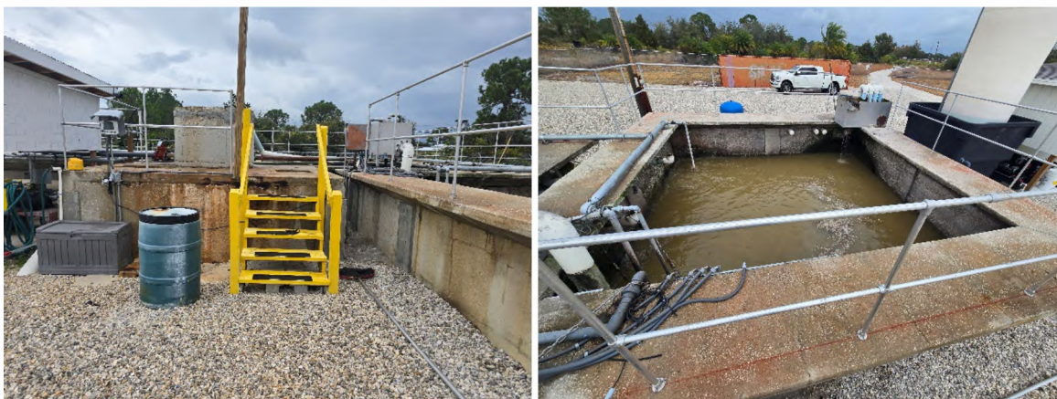
New access stairs with handrails, high friction tread plates, high visibility coating (left) and new fall protection rails around the exterior of the facility to prevent falls from the plant (right).
