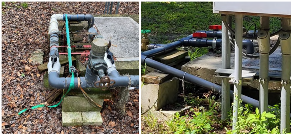
Improper repairs to discharge piping at main lift station with PVC and ratchet straps (left) and new discharge piping (right)
