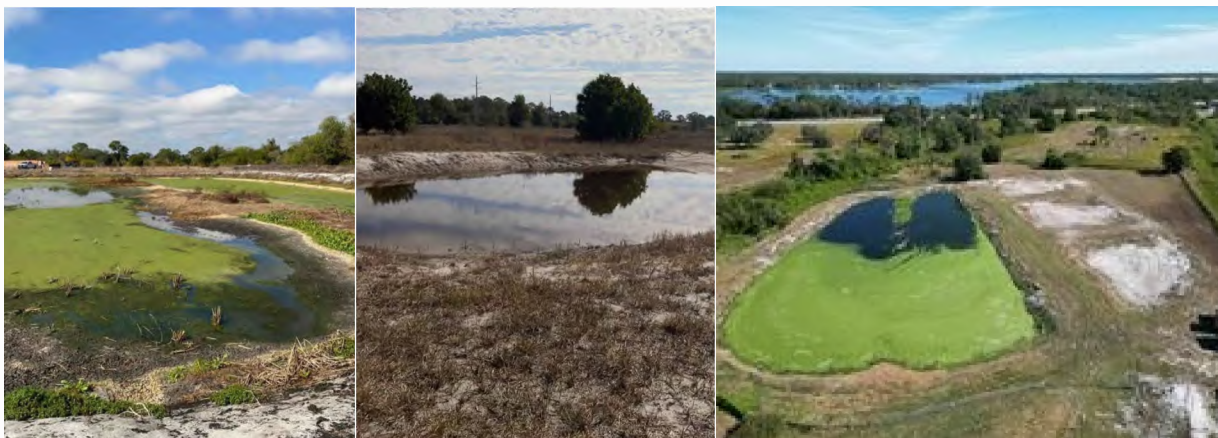
17 Rapid infiltration basin (left) and percolation ponds (center) before sludge and vegetation 18 removal. Note percolation pond is holding water rather than draining both due to 19
