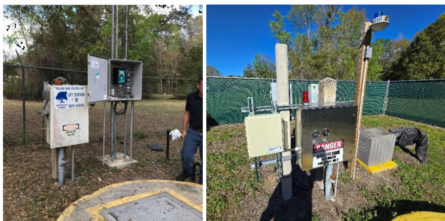
Example of before (left) and after (right) control panel replacement at Lift Station #9. Note remote monitoring unit to the left of the new panel installed as well to be discussed below.
