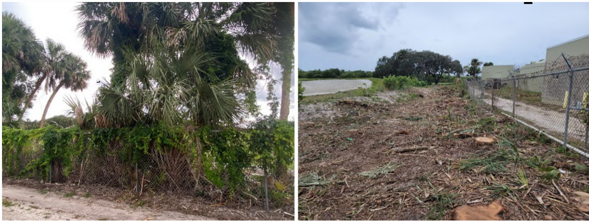
Clearing of vegetation from facility fence line
