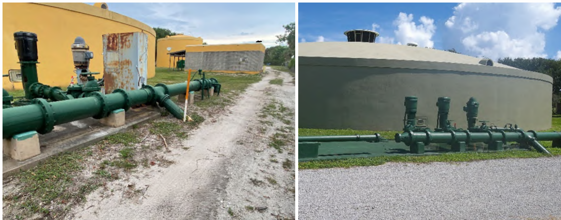
Before (left) and after (right) access road improvements and piping and equipment recoating.
