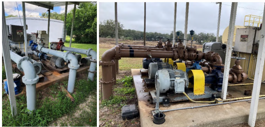
Examples of before (left) and after (right) recoated piping and equipment (effluent pumps and piping)
