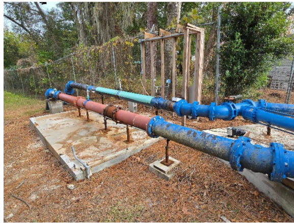
Replaced segment of above ground piping
