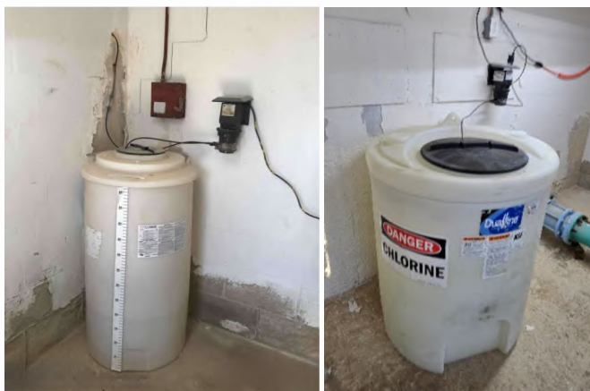
Example of sodium hypochlorite drums before (left) and after (right) replacement in this cast at Well 6.
