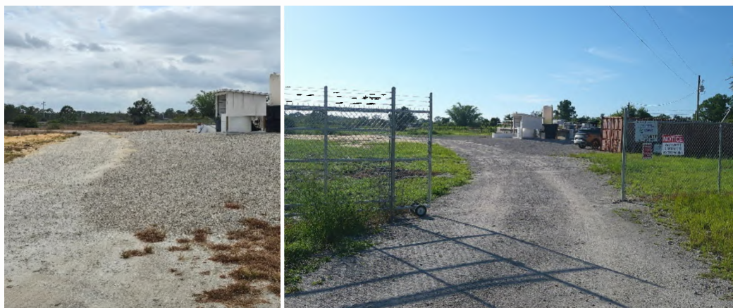
Site and road conditions following improvement.
