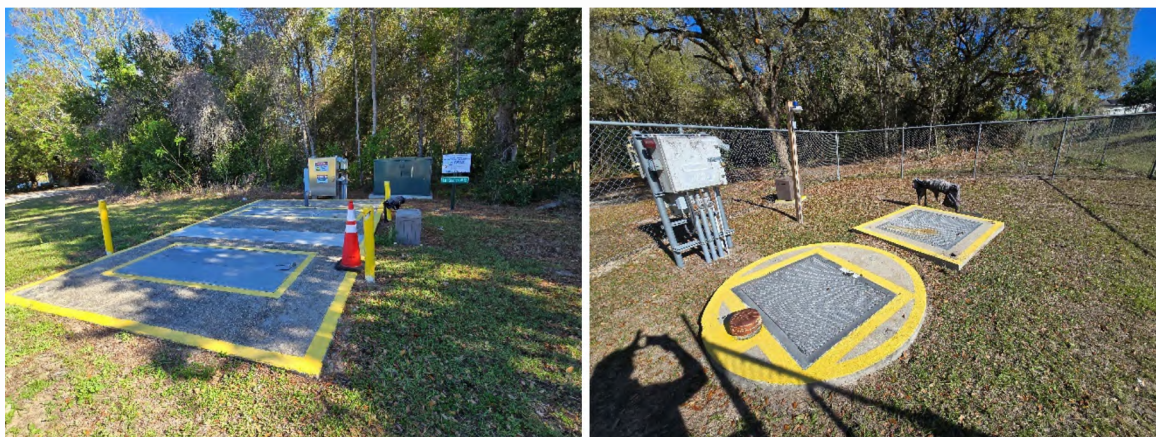
Examples of high visibility paint application to tripping hazards.
