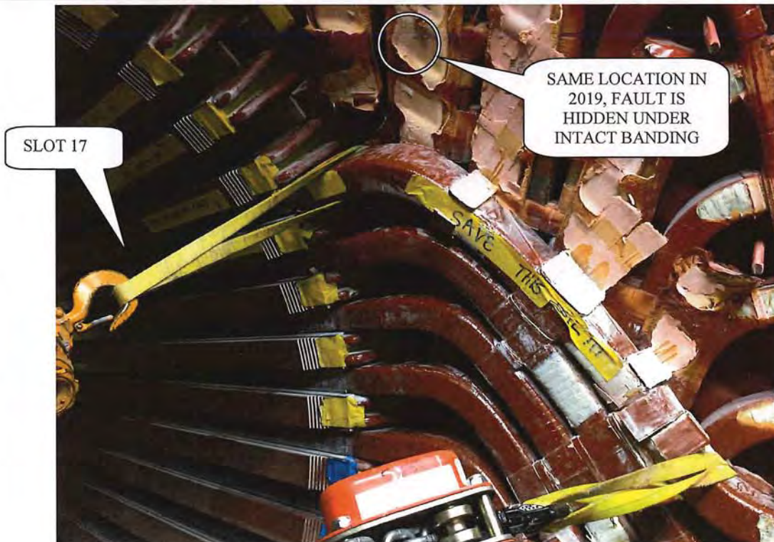
May 2019 - Removal of Top Bar in Slot 17.
