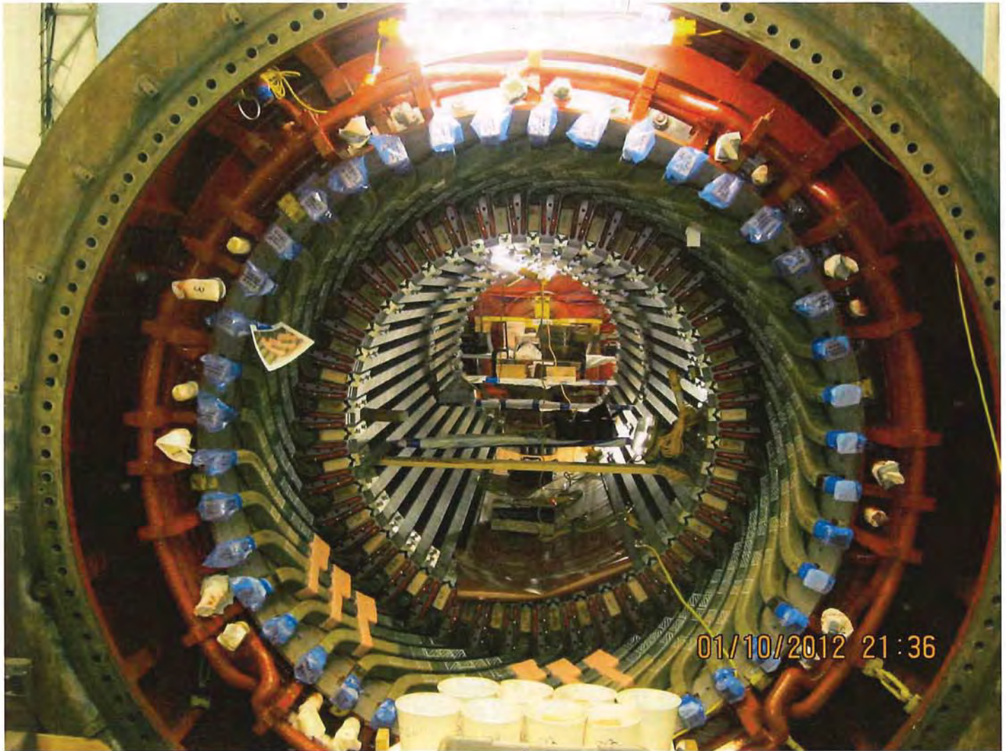
Figure 2 – Bottom Half-Coil installation
