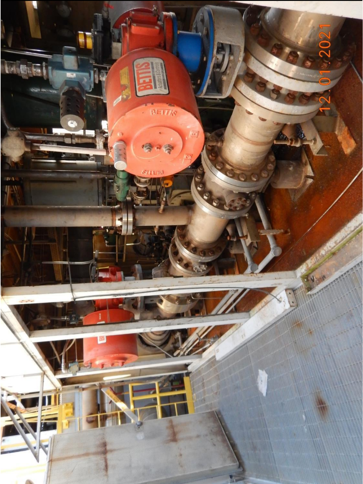
Syngas Line showing both Syngas block valves and control valves
