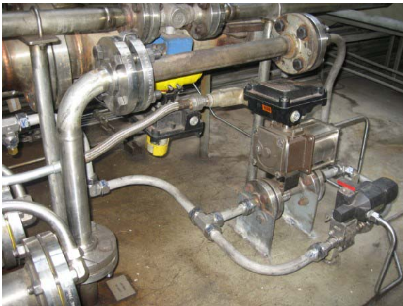
Purge Valve Re Located
