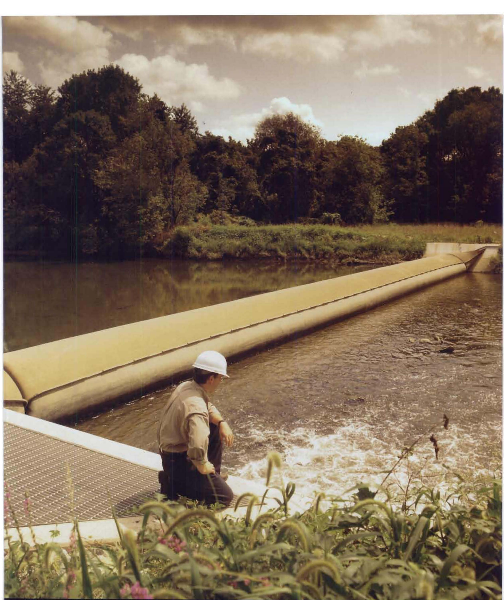
Located near Wilmington, Delaware, this inflatable rubber dam exemplifies United Water's historic role as a technological innovator. The dam, which can be inflated to capture fresh water and deflated to return the stream to its normal flow, is the first to be used in North America to ensure a drinking water supply.
