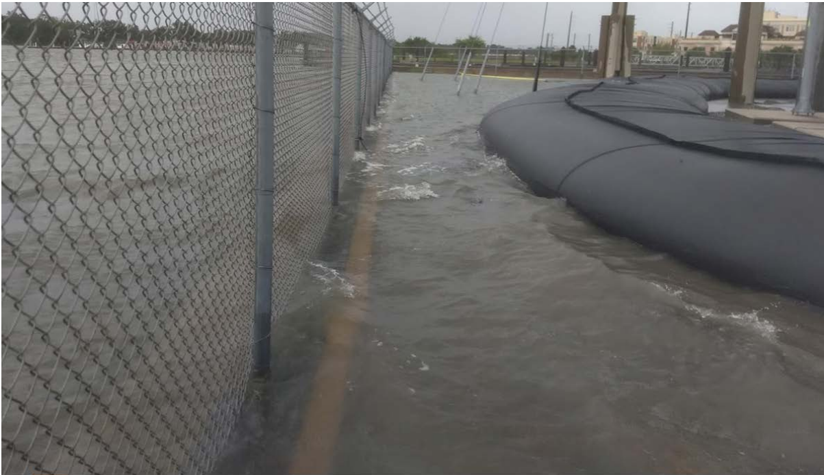
St. Augustine AquaDam during hurricane at high tide
