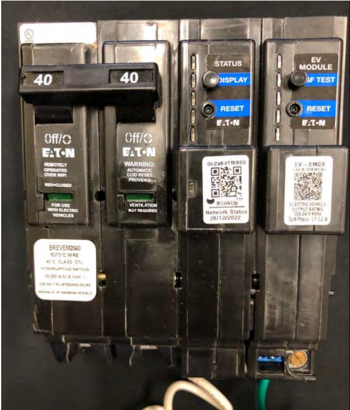
Figure 3 Electric Vehicle version of the EMCB. Note that it takes a total of four slots for this two-pole device.
