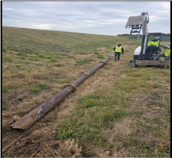
SDT-1 Buried Drain Line Removal
