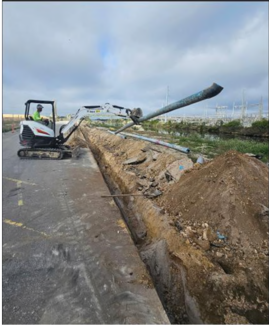
SDT-1 Buried Drain Line Removal
