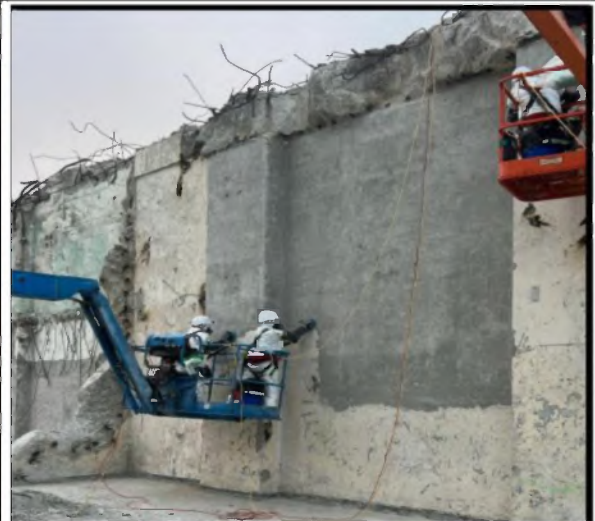
Power Block – Decon Wall paint Removal
